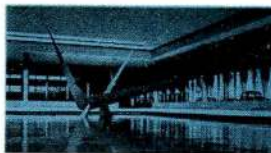
Ottawa Air Terminal Architects, Gilleland and Strutt, Ottawa; Sculpture by Louis Archambault
