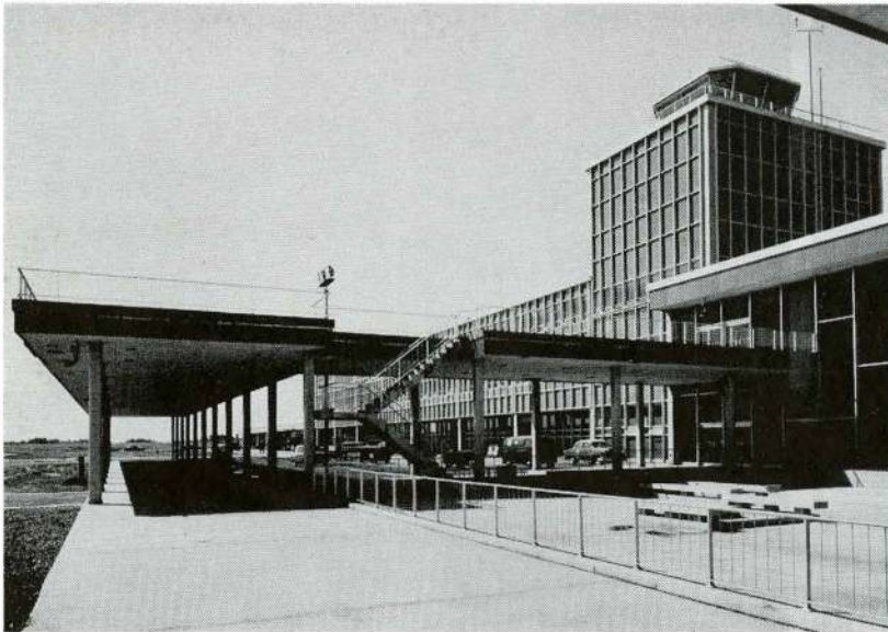
View of spectators' deck from tarmac
