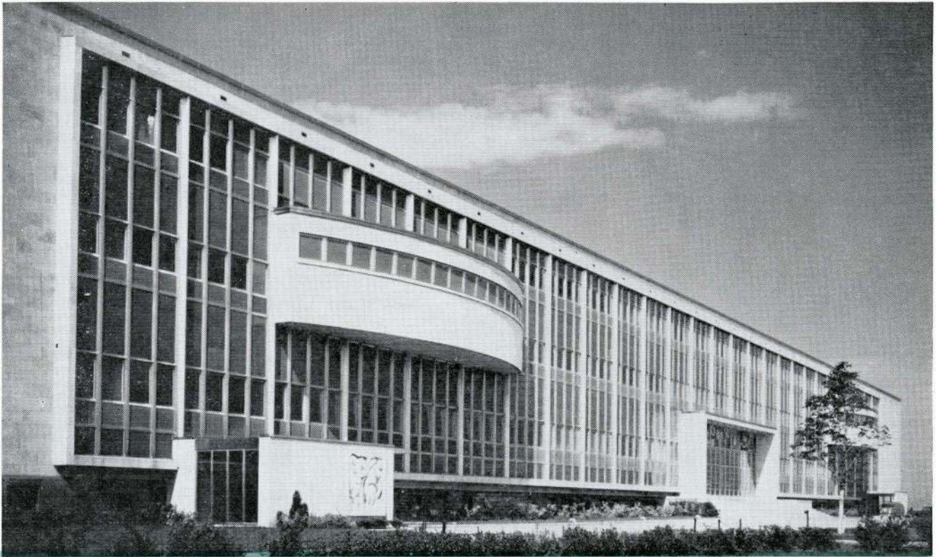
New Laval University Medical School in Quebec City is designed with nickel stainless steel kalamein curtain walls fabricated by National Window Company Ltd., Montreal. Architect: Lucien Mainguy, Quebec City.
