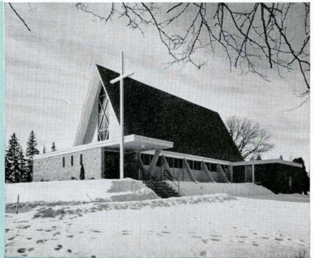
Nickel stainless steel mullions lend bright beauty to St. George's Roman Catholic Church in Byron, Ontario. Fabricator: Macotta Company of Canada Limited. Architects: Blackwell and Hagarty.
