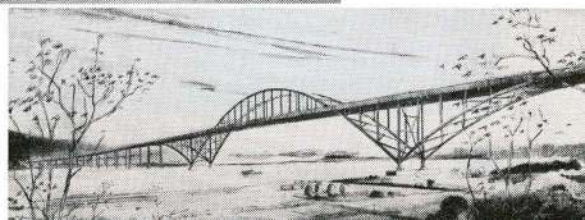
Port Mann (under construction)
