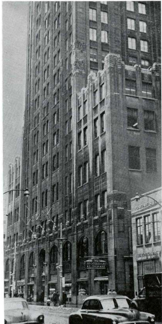
Toronto Star Building Consulting Engineer, R. T. Tamblin & Partners Ltd. Mechanical Contractor, Universal Plumbing & Heating Ltd.
