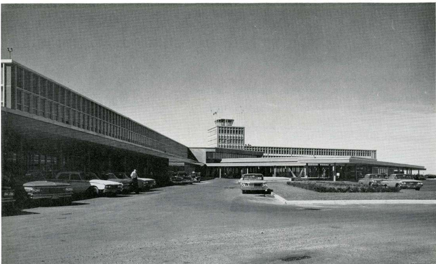
Ottawa: General view of building showing porte-cochere and main entrance
