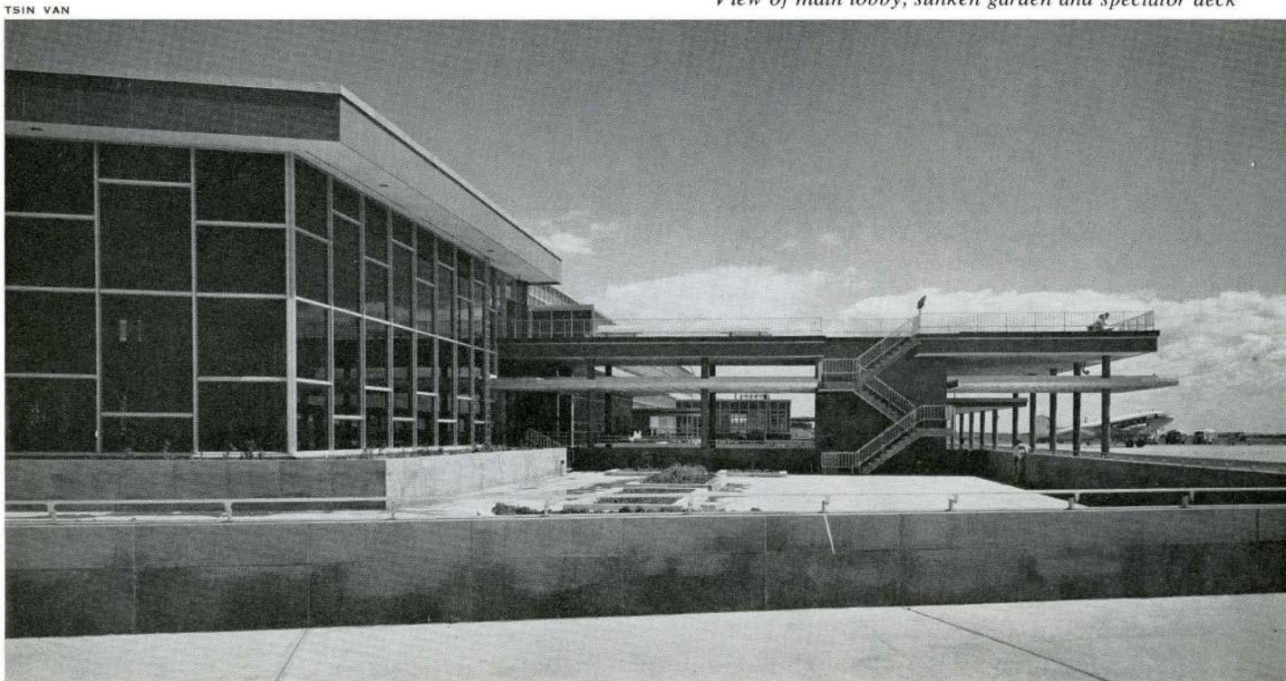
View of main lobby, sunken garden and spectator deck
