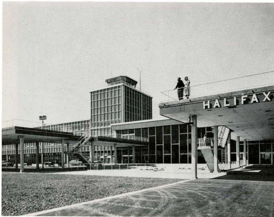
Left: view of sunken garden, main lobby and spectators' deck from tarmac
