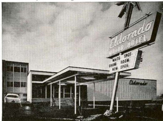
THE ELDORADO is modern to the "nth" degree. This split-level establishment was designed by Architect H. N. Semmens, Fred Welsh & Son Ltd., Mechanical Contractors.
