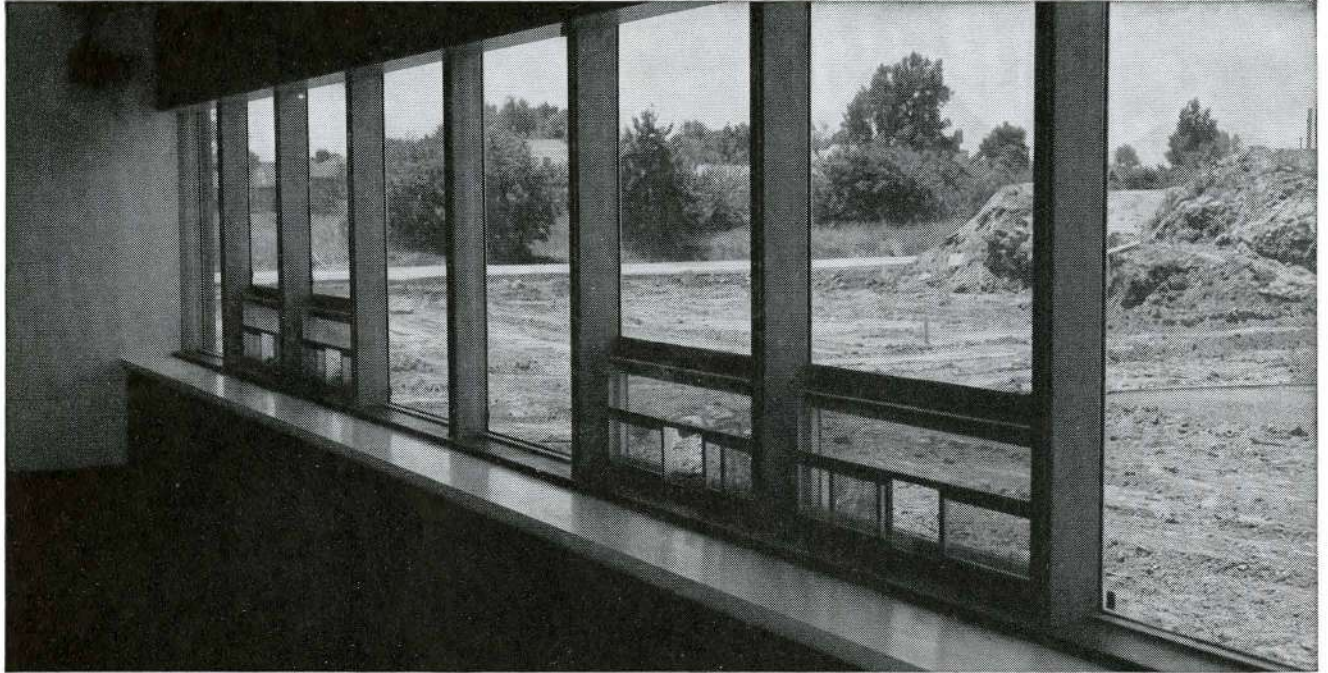
Anna Merritt Elementary School, Lockport, New York, covers an area of 17,111 sq. ft., features a new aluminum framing system with a neoprene seal that eliminates caulking.
