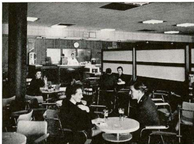
IN THE BEVERAGE ROOM a Honeywell Electronic Air Cleaner removes tobacco smoke and other impurities. Honeywell's Electronic Air Cleaner removes 6 times more dirt than ordinary filters.
