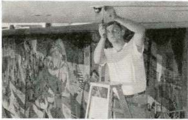
Smartly styled, unobtrusive Edwards automatic fire detectors are located throughout the theatre—even in the muralled main lobby.
