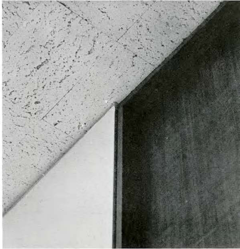
Detail at head of door and ceiling
