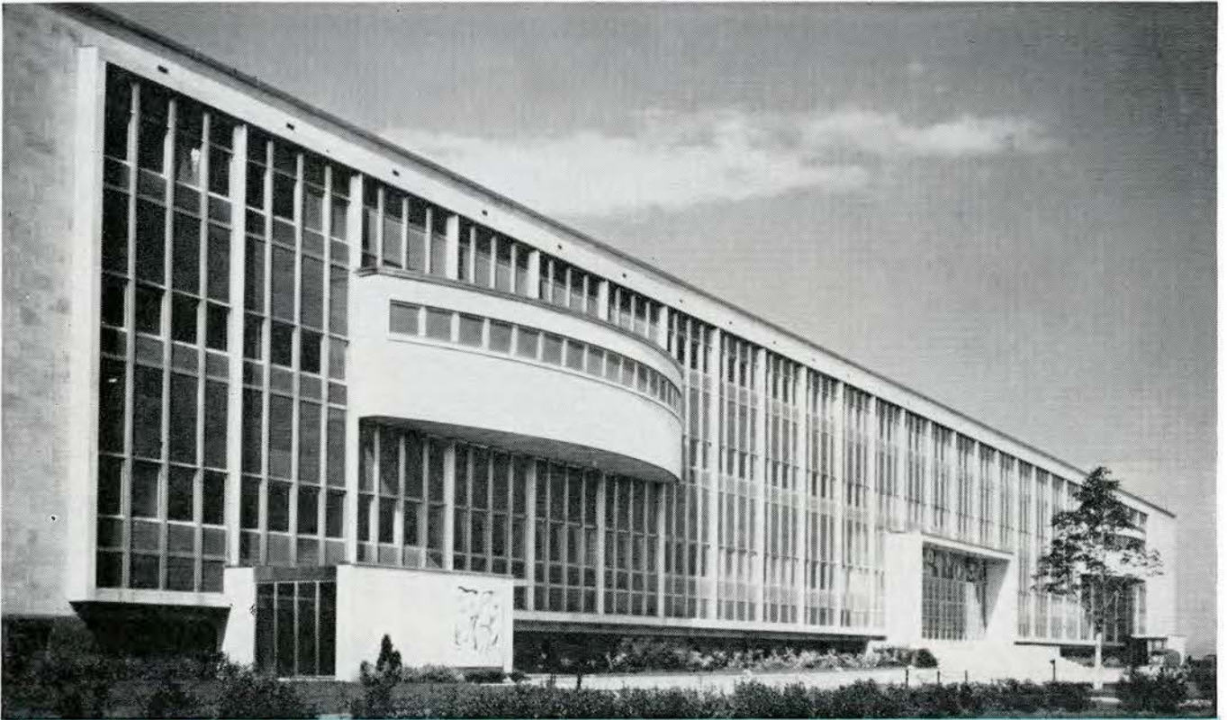
New Laval University Medical School in Quebec City is designed with nickel stainless steel kalamein curtain walls fabricated by National Window Company Ltd., Montreal. Architect: Lucien Mainguy, Quebec City.
