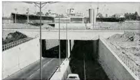
DEAS ISLAND TUNNEL
