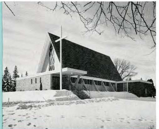
Nickel stainless steel mullions lend bright beauty to St. George's Roman Catholic Church in Byron, Ontario. Fabricator: Macotta Company of Canada Limited. Architects: Blackwell and Hagarty.
