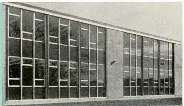
Nickel stainless steel curtain wall at Oakridge Senior Public School, St. Catharines, Ontario. Fabricator: Macotta Company of Canada, Limited. Architects: Salter and Flemming.
