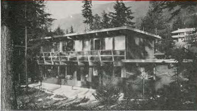
771 Winona, North Vancouver, British Columbia. Builder: Lewis Construction Co. Ltd., West Vancouver, B.C.
