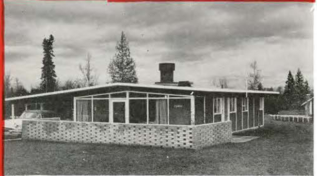
21025 Maple Ave., Langley, British Columbia. Builder: Dodd Construction Ltd., P.O. Box 715, Langley, B.C.
