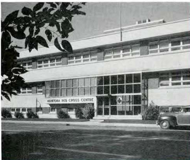
Entranceway and windows of new Manitoba Red Cross Centre on Osborne St., Winnipeg, are of nickel stainless steel. Fabricator: Dominion Bronze and Iron Ltd., Winnipeg. Architects: Moody and Moore, Winnipeg.
