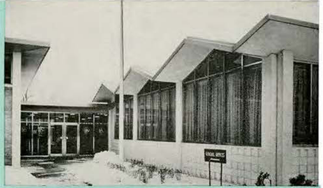
New office building of Parke, Davis & Company, Ltd. in Montreal features nickel stainless steel window walls and entranceway fabricated by Canadian Pittsburgh Industries Limited of Montreal. Architect: Paul H. Lapointe. Engineer: R. P. Steketee, c/o Giffels & Vallet of Canada, Ltd.
