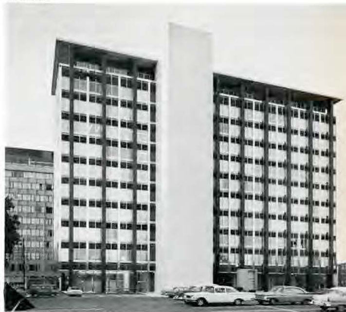
South elevation, showing elevator tower and circular service elevator shaft.
