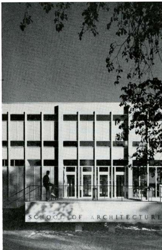
The entrance of the School of Architecture building at the University of Manitoba is shown here. Quality of pre-cast concrete is clearly visible. Architects and engineers for the project were Smith, Carter, Searle Associates; general contractor, North American Building Ltd.
