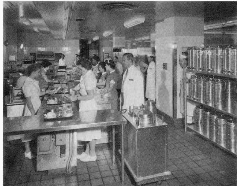
Kitchen, showing double service line
