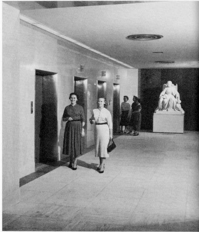
Main Entrance, Elevator Lobby, Surgical Wing
