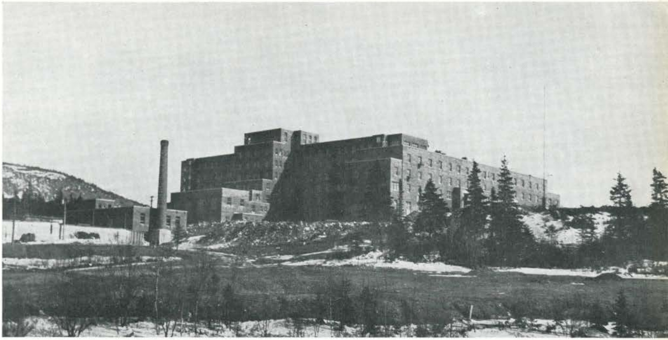
REAR VIEW SHOWING RESIDENCE TO THE RIGHT
