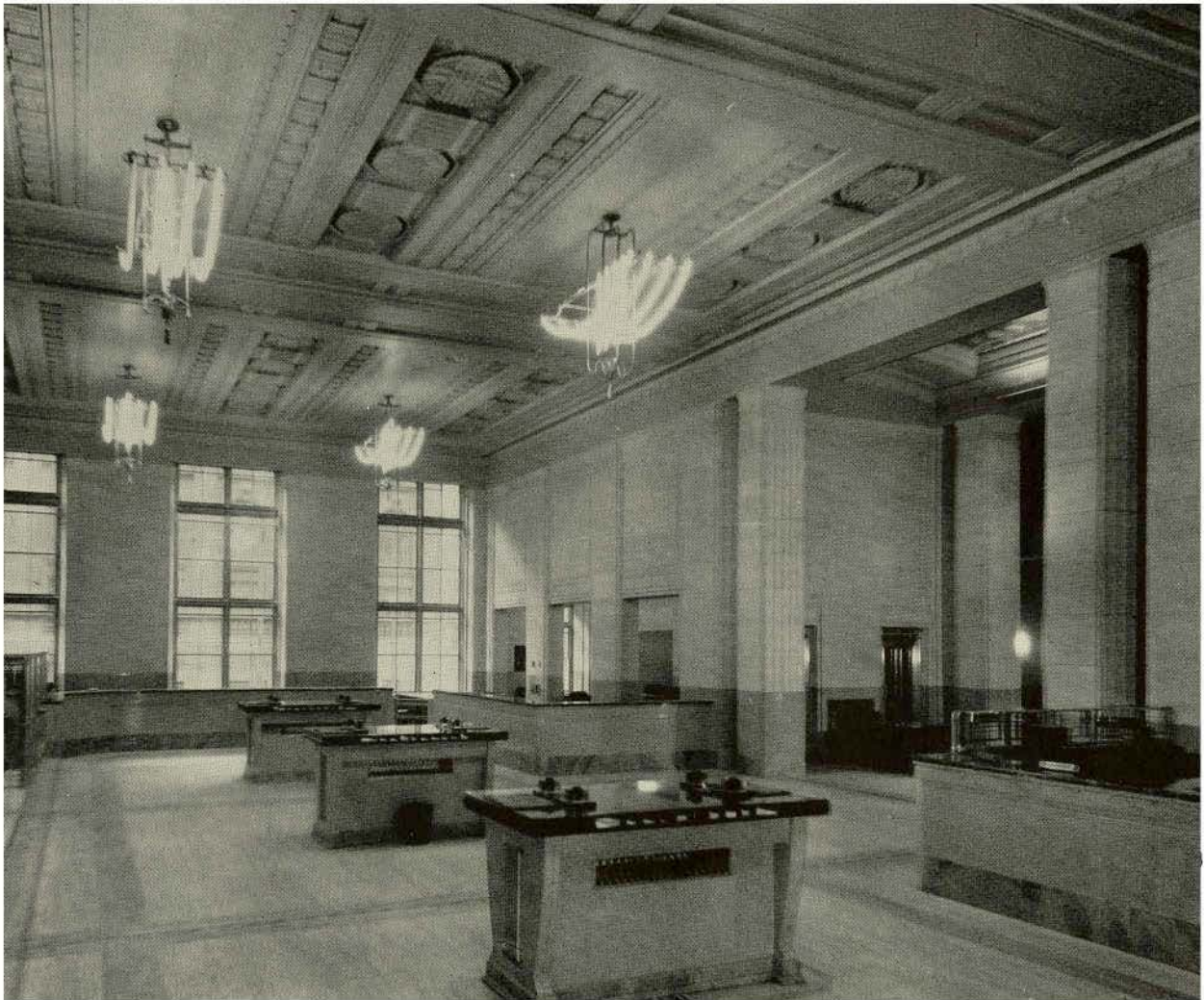
BANKING ROOM—IMPERIAL BANK BUILDING, TORONTO Sproatt & Rolph, Architects
