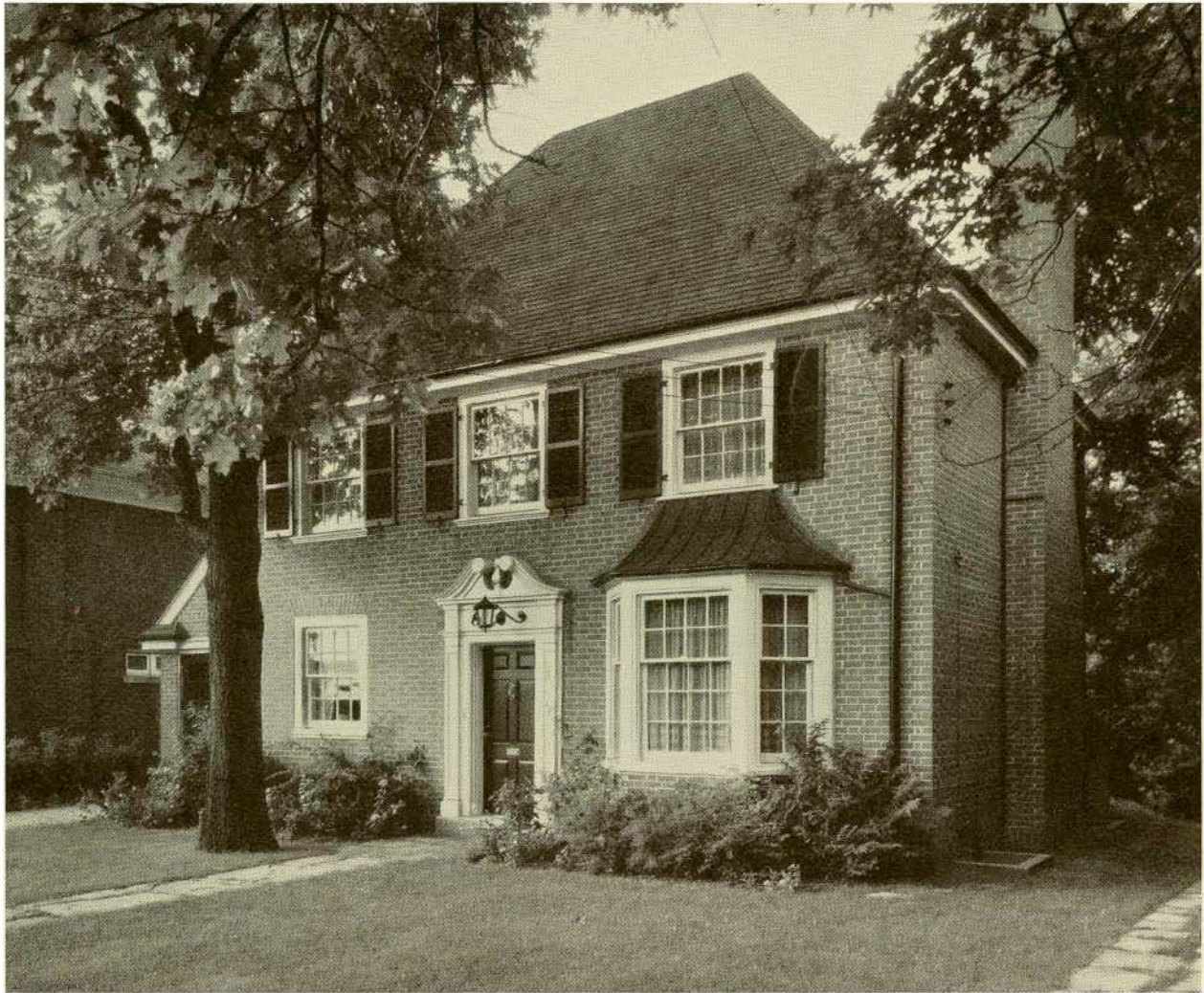
RESIDENCE AT SWANSEA, ONT.
