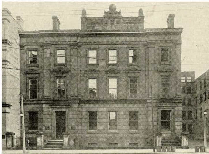
THE COMMERCIAL BANK, WELLINGTON STREET, TORONTO, (1845) NOW OCCUPIED BY MESSRS. CLARKSON, GORDON, DILWORTH, GUILFOYLE AND NASH
