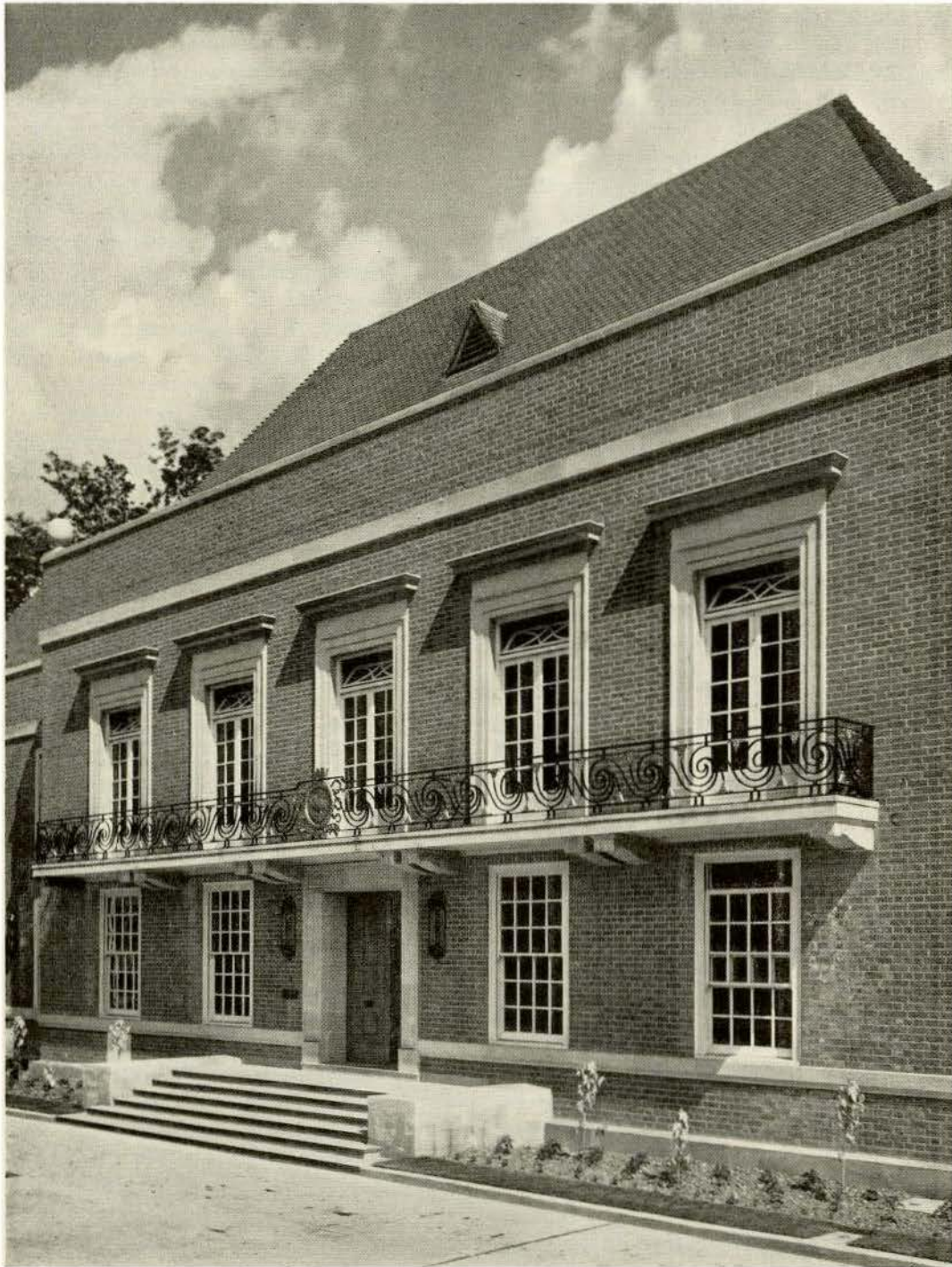
ENTRANCE DETAIL MUNICIPAL OFFICES—HIGH WYCOMBE, ENGLAND
