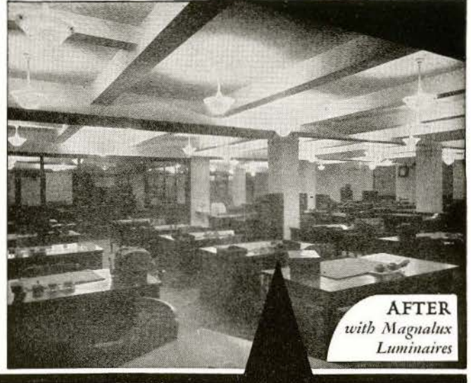
Both installations use the same wattage lamps. Absence of glare and good light distribution is to be noted in the illustration on the right.
