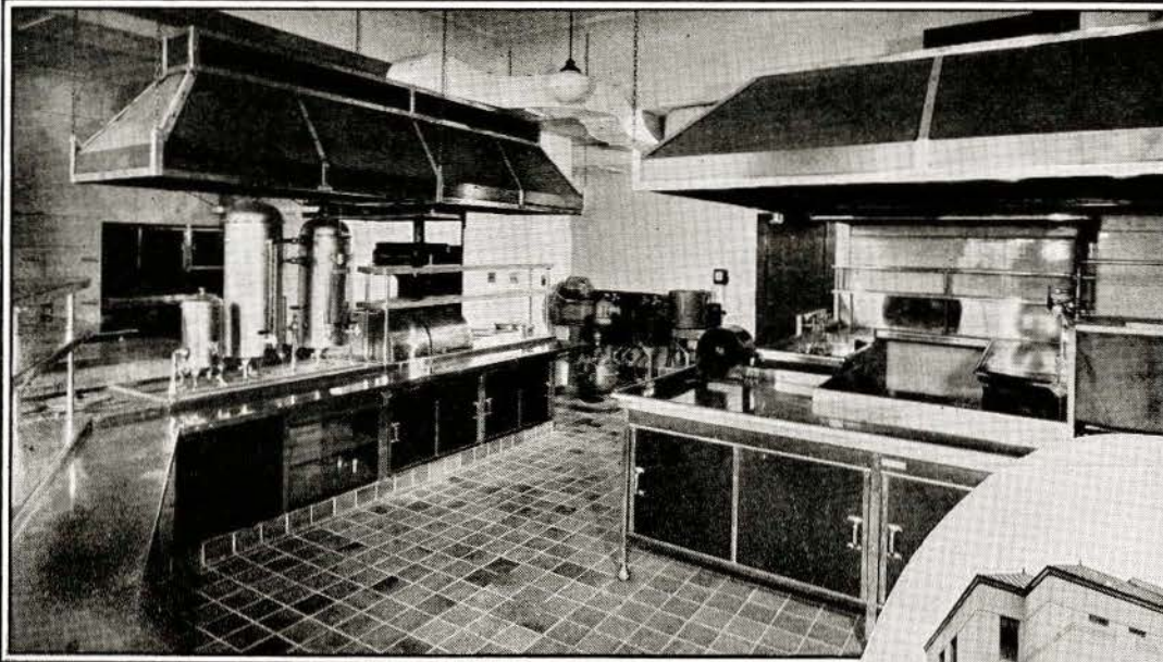
Cafeteria and kitchen in North American Life Assurance Company Head Office Building, showing Monel Metal equipment.
