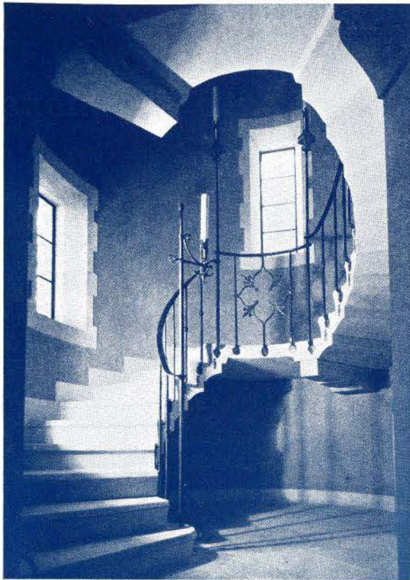
AN INTERESTING MODERN APPLICATION OF CUT STONE CIRCULAR STAIRCASE IN RESIDENCE OF A. H. C. PROCTOR, ESQ. HUGH L. ALLWARD, ARCHITECT STONE WORK BY NICHOLSONS
