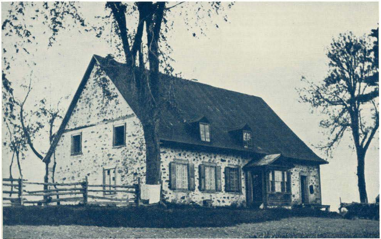
THE SOUTH SIDE BEFORE RESTORATION
