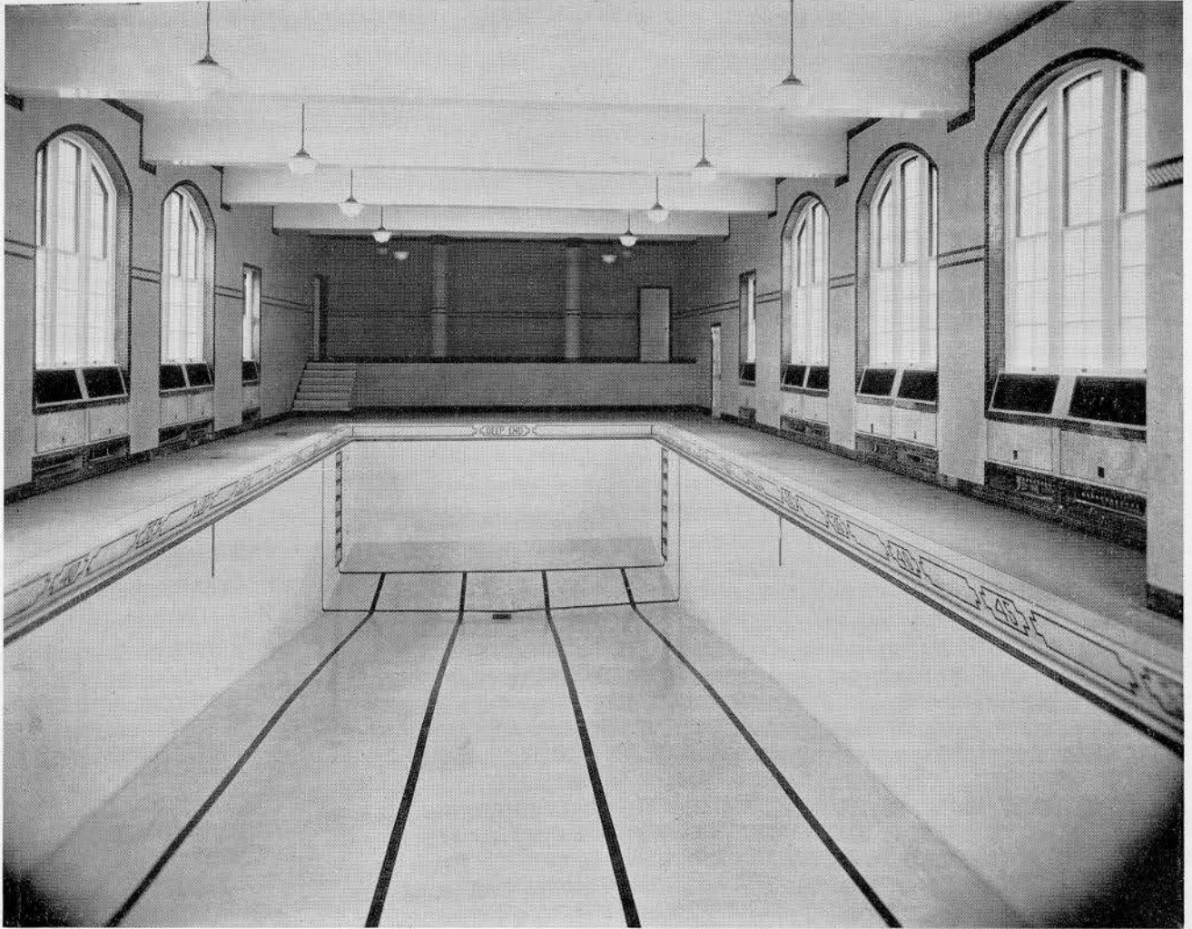
THE CERAMIC MOSAIC TILED SWIMMING POOL IN THE LORD BEAVERBROOK RESIDENCY, FREDERICTON, N.B. Architects: MESSRS. ALWARD & GILLIES, ST. JOHN
