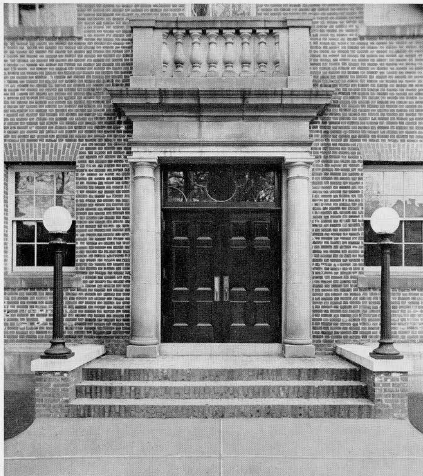
DETAIL OF MAIN ENTRANCE
