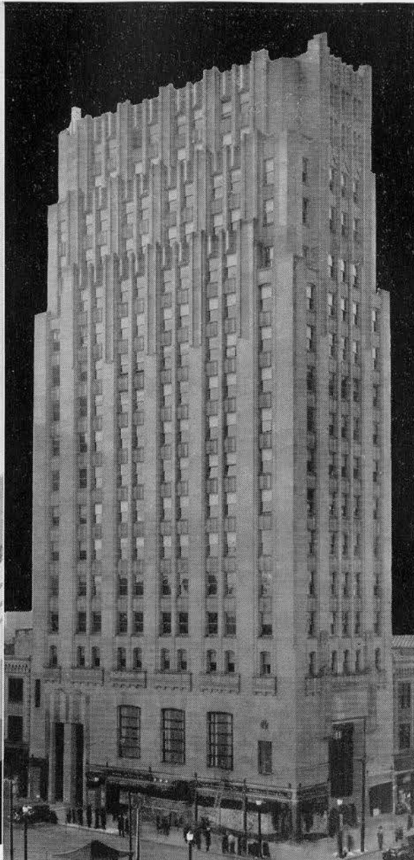
Central Tower . . . . . Youngstown, Ohio Morris W. Scheibel, Architect . . . . . W. J. Scholl Co., Heating Contr.
