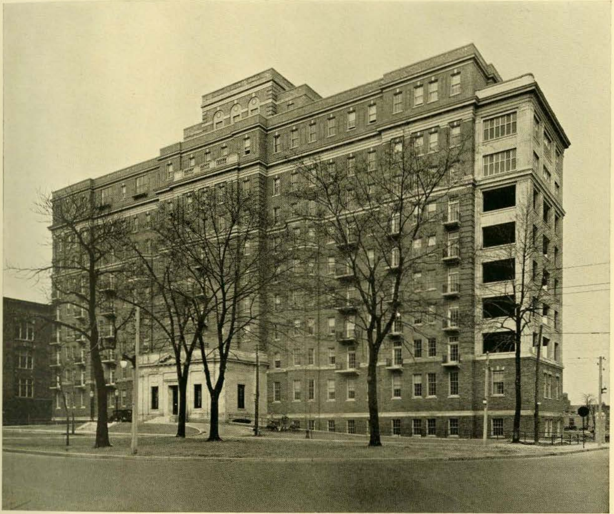
NEW PRIVATE PATIENTS' PAVILION, TORONTO GENERAL HOSPITAL Darling & Pearson, Architects
