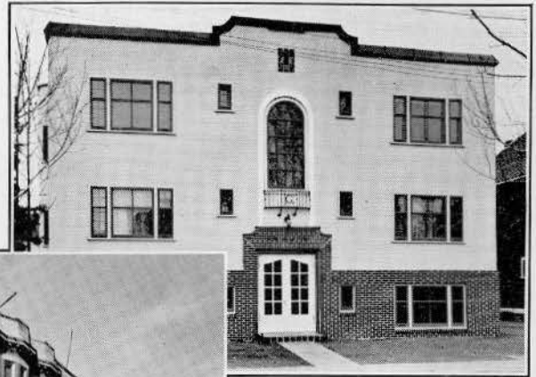
The Garden Apartments, 14th Avenue, West, Calgary, Alta. Twelve suites - all equipped with Frigidaire.
