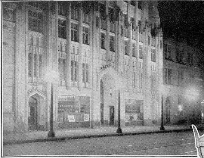
Pigott Building, James St., Hamilton, Illuminated by Westinghouse Duolux Lighting Units.
