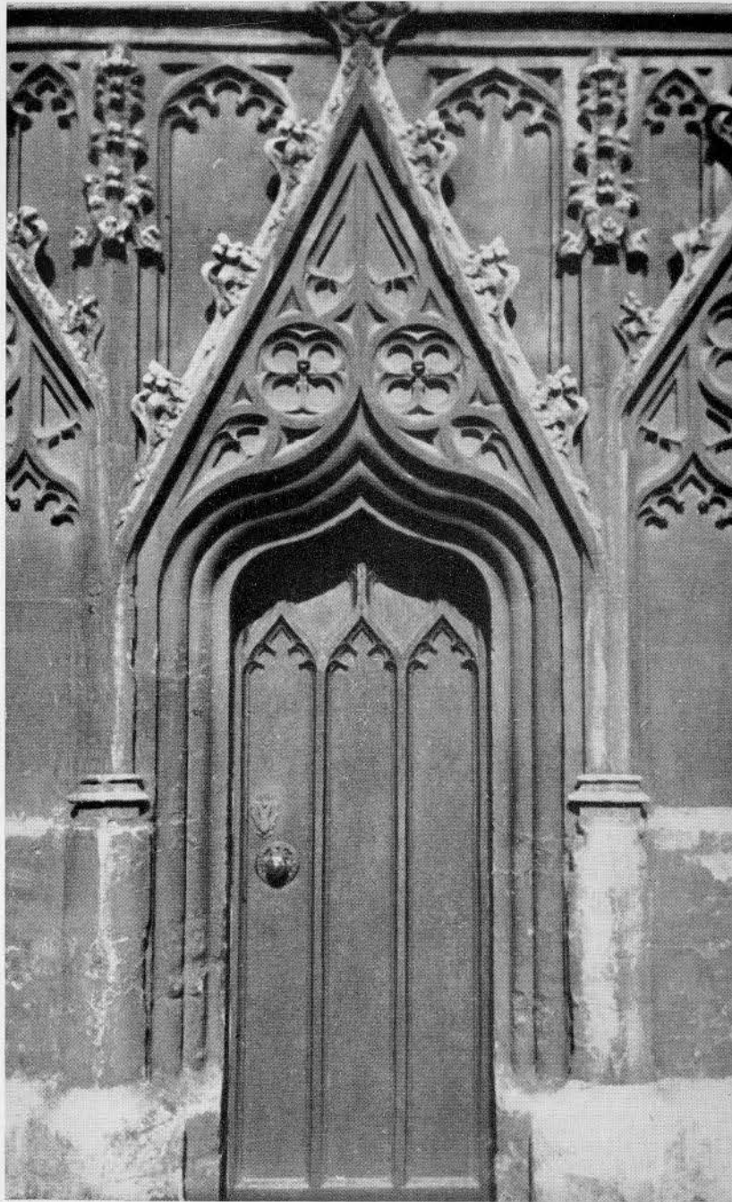
DOORWAY—ST. MARY REDCLIFFE, BRISTOL, ENGLAND
