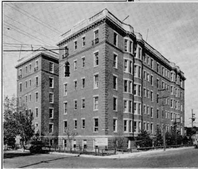
Anderson Apartments 18th Avenue and 7th Street, West Calgary, Alta. All sixty suites equipped with Frigidaire.
