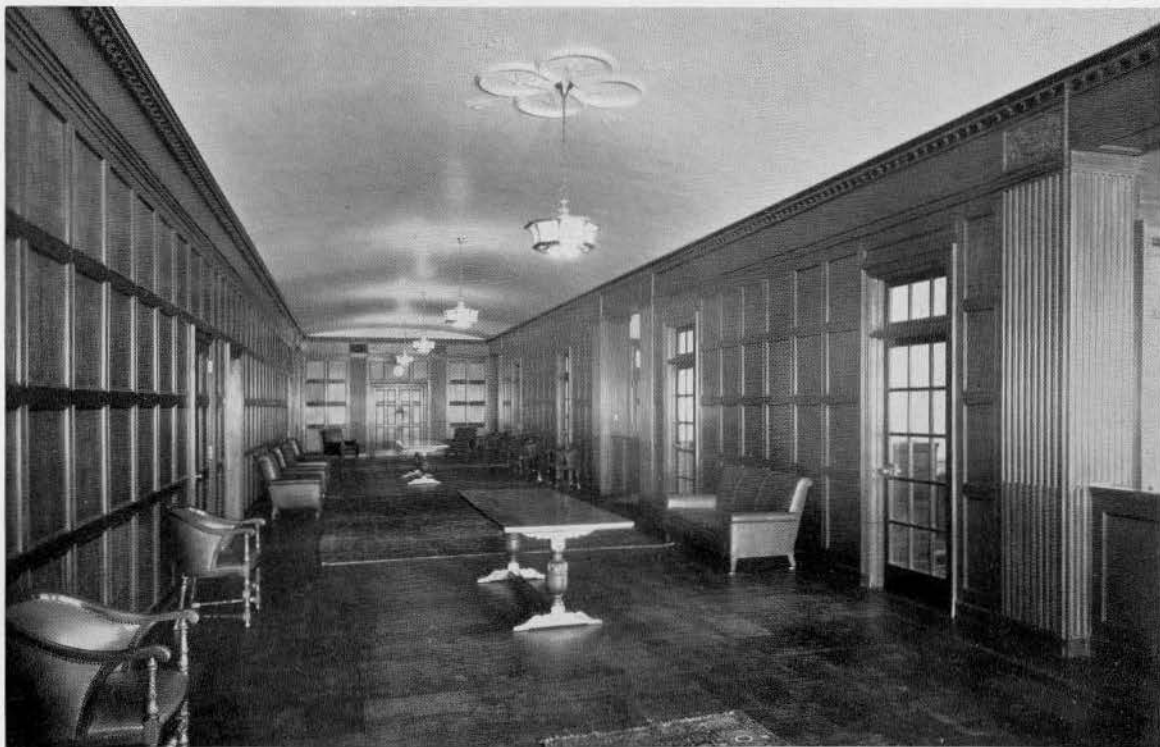
RECEPTION HALL ON SEVENTEENTH FLOOR
