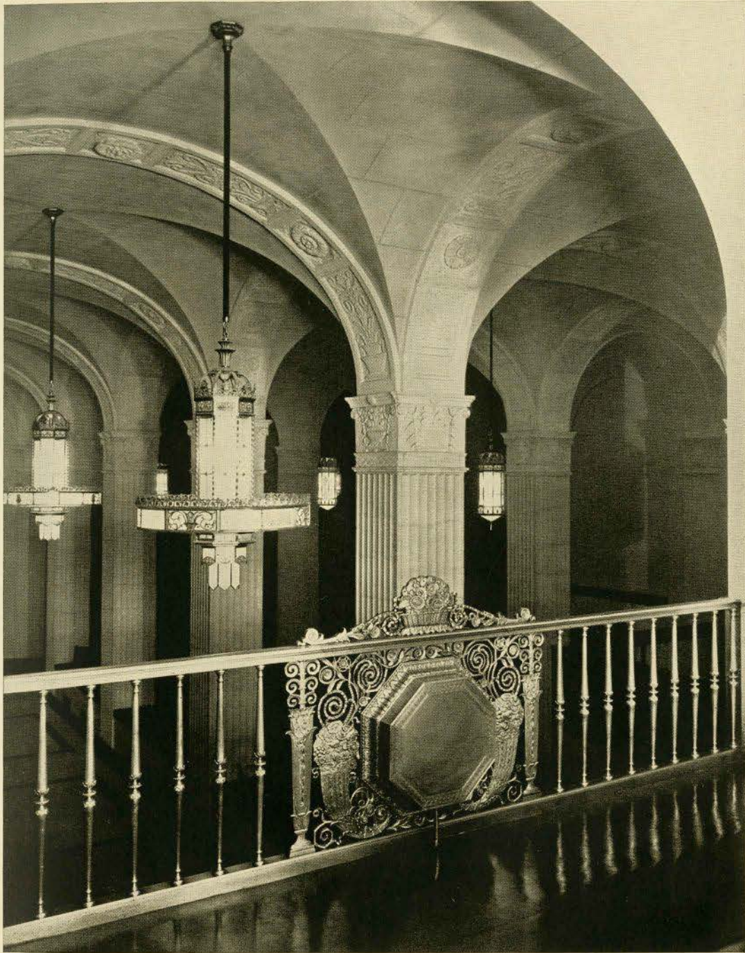
DETAIL OF BANKING ROOM FROM MEZZANINE CANADA PERMANENT BUILDING, TORONTO
