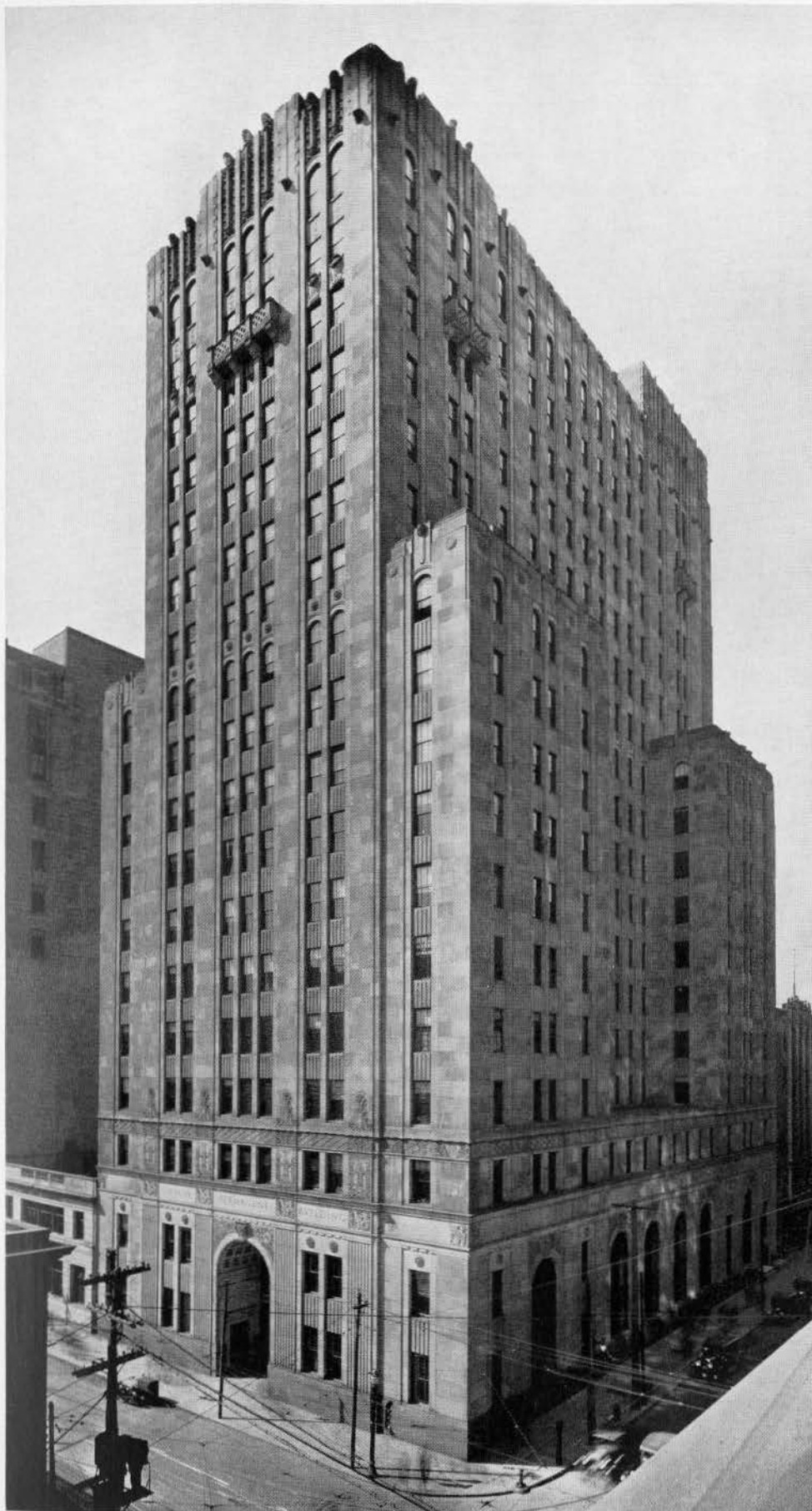
CANADA PERMANENT BUILDING, TORONTO, View from North-east
