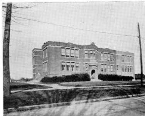
VICTORIA SCHOOL, ST. CATHARINES, ONT. Walls and Ceilings were decorated with Walpamur under the direct supervision of C. W. McBride Secretary of the Board of Education
