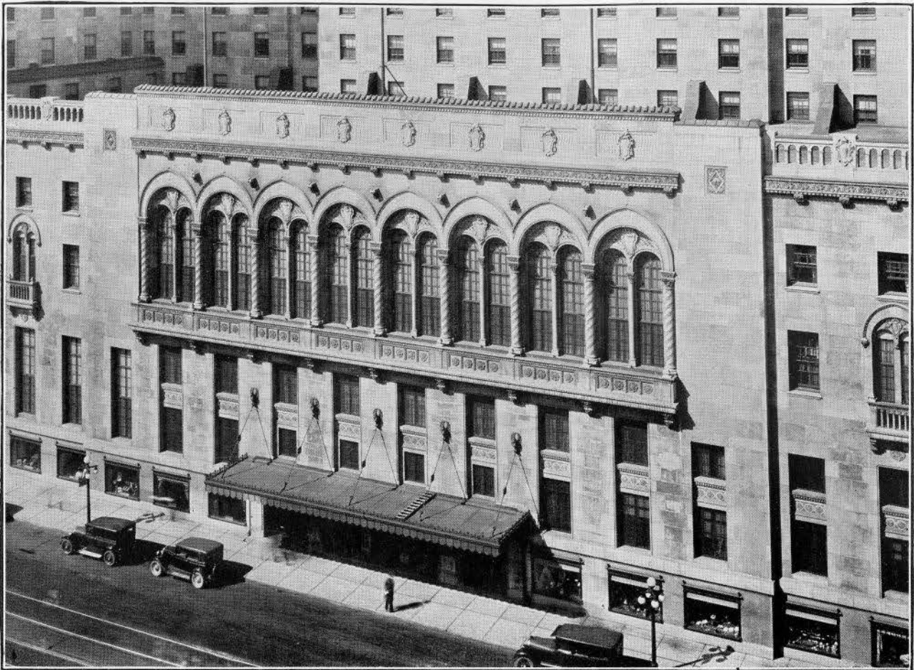
Detail, Royal York Hotel, Toronto. Ross & MacDonald, Architects. Sproatt & Rolph, Associate Architects. Anglin-Norcross Company, Builders. ILCO "Dark Hollow" Variegated Indiana Limestone
