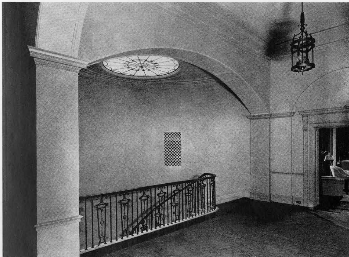
STAIR HALL ON SECOND FLOOR
