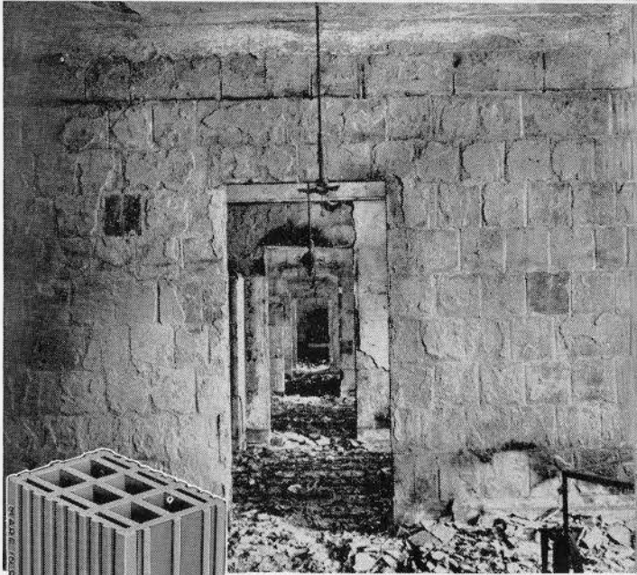
SPRING VALLEY WATER WORKS BUILDING Showing Endurance of Clay Tile
