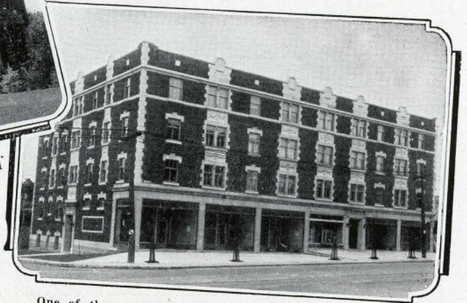
One of three apartment houses erected by Kaufman Construction Co., Northcliffe Ave. and Sherbrooke St., Montreal. Celotex Lath used as plaster base.
