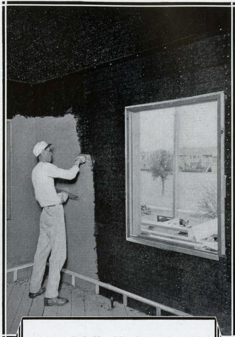
Armstrong's Corkboard Insulation on the second floor of Mr. H. B. Thompson's residence at Dallas, Texas. The plaster is being applied directly on the cork, without lath.
