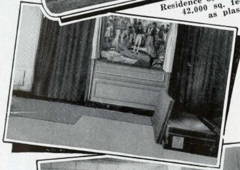
Lord Nelson Hotel, Halifax. Celotex used as carpet lining.
