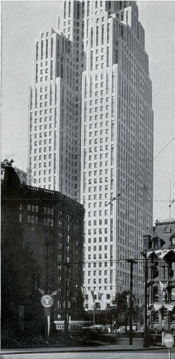
The Penobscot Building, Detroit
