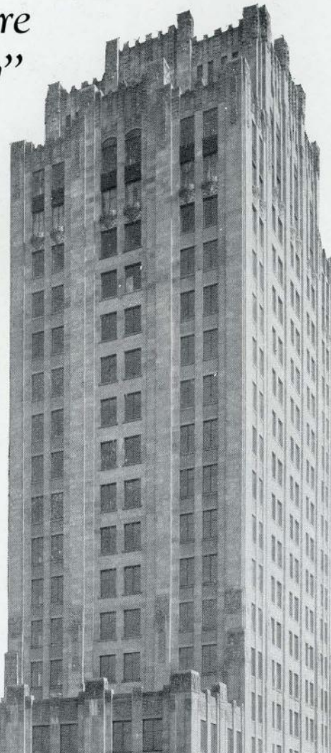
Toronto Daily Star Building, Toronto, Canada. Chapman & Oxley, Architects. Thompson-Starrett Co., Builders. First two stories Canadian granite; other 20 stories Standard Gray Indiana Limestone.
