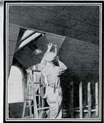
The cork-lined home of Mr. William P. Fosdick, Cincinnati, Ohio. Charles F. Cellarius, architect.
