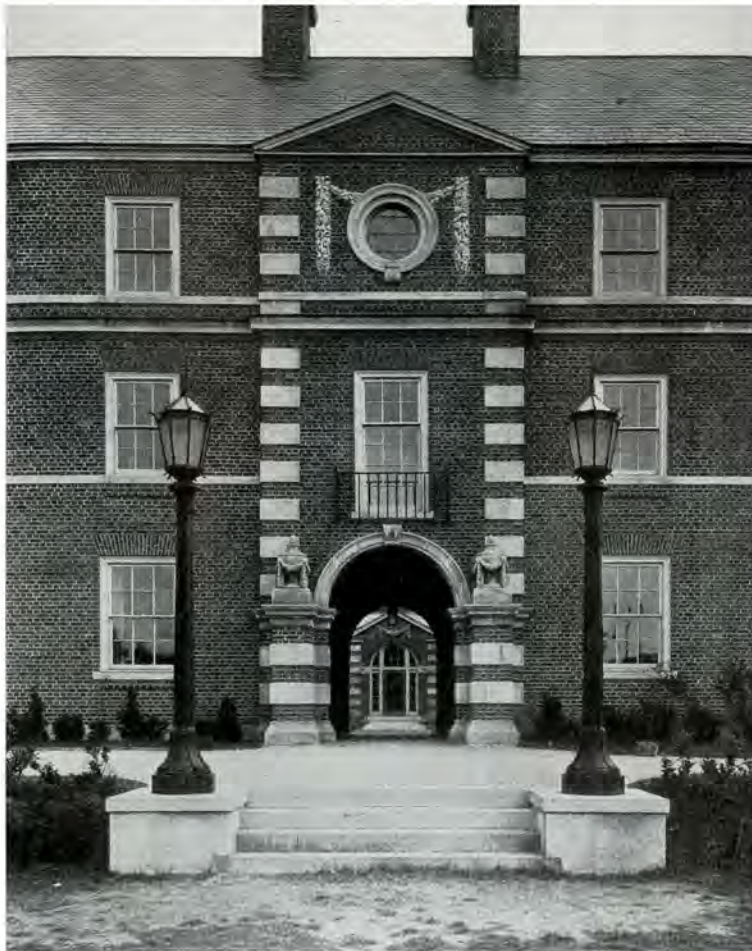
ONE OF THE ARCHES TO QUADRANGLE LOWER SCHOOL, RIDLEY COLLEGE, ST. CATHARINES, ONT. Marani, Lawson and Paisley, Architects
