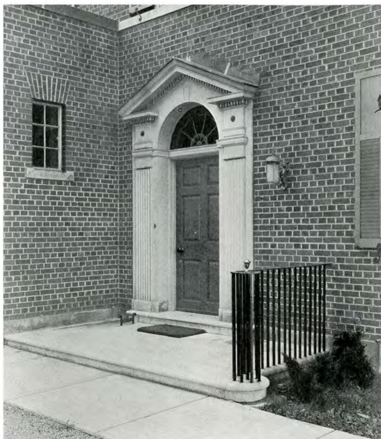
ENTRANCE DOOR—PRINCIPAL'S RESIDENCE
