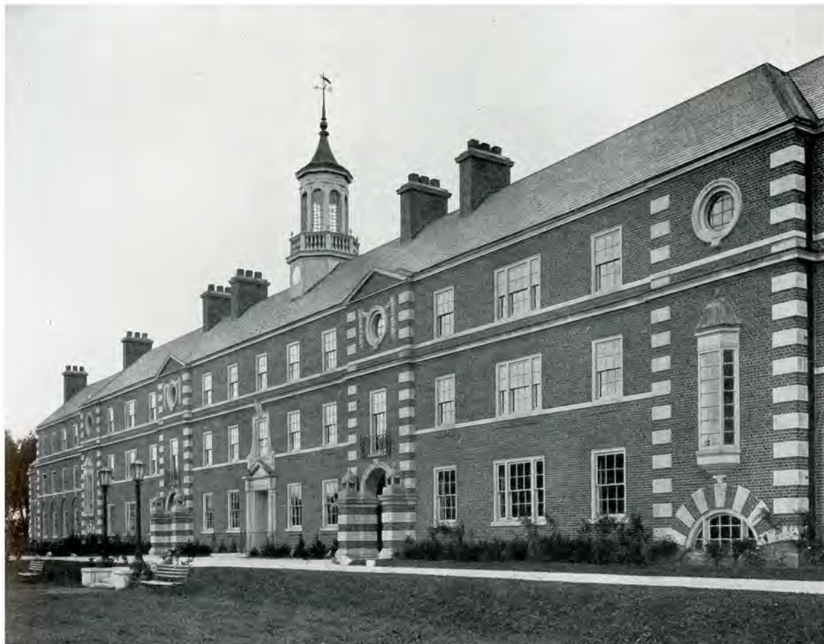
LOWER SCHOOL, RIDLEY COLLEGE—VIEW FROM THE PLAYING FIELD Marani, Lawson and Paisley, Architects
