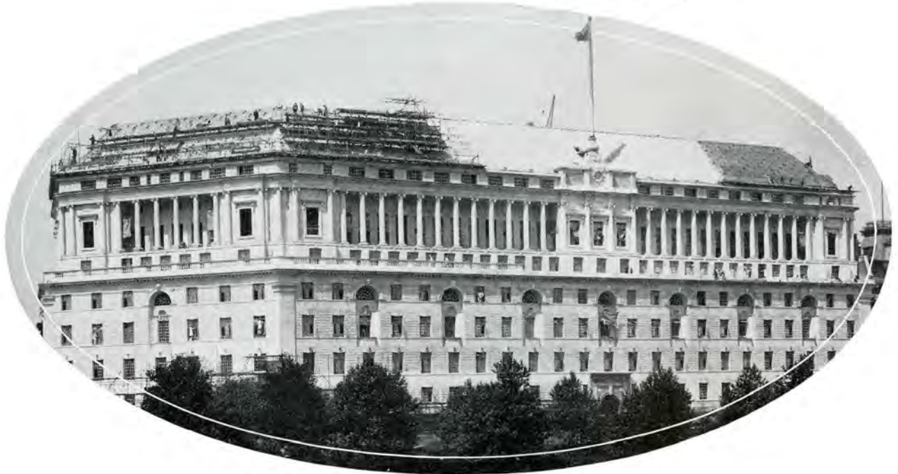
Industry House—Imperial Chemical Industries Ltd., Millbank, London, England— Equipped with 20,000 feet of Vita Glass.
