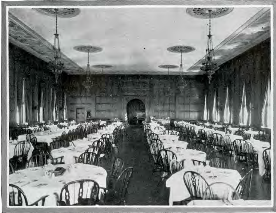
Johns-Manville Sound-absorbing Treatment on the ceiling of this dining room at the Cincinnati Chamber of Commerce subdues unnecessary noise. Tietig & Lee and Harry Hake, Architects
