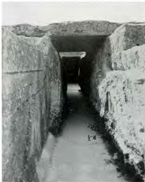
THE DEPOSIT LINING THE WATER CONDUIT
