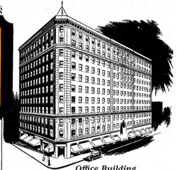
Office Building Plumbing, Heating and Sprinkler Systems
