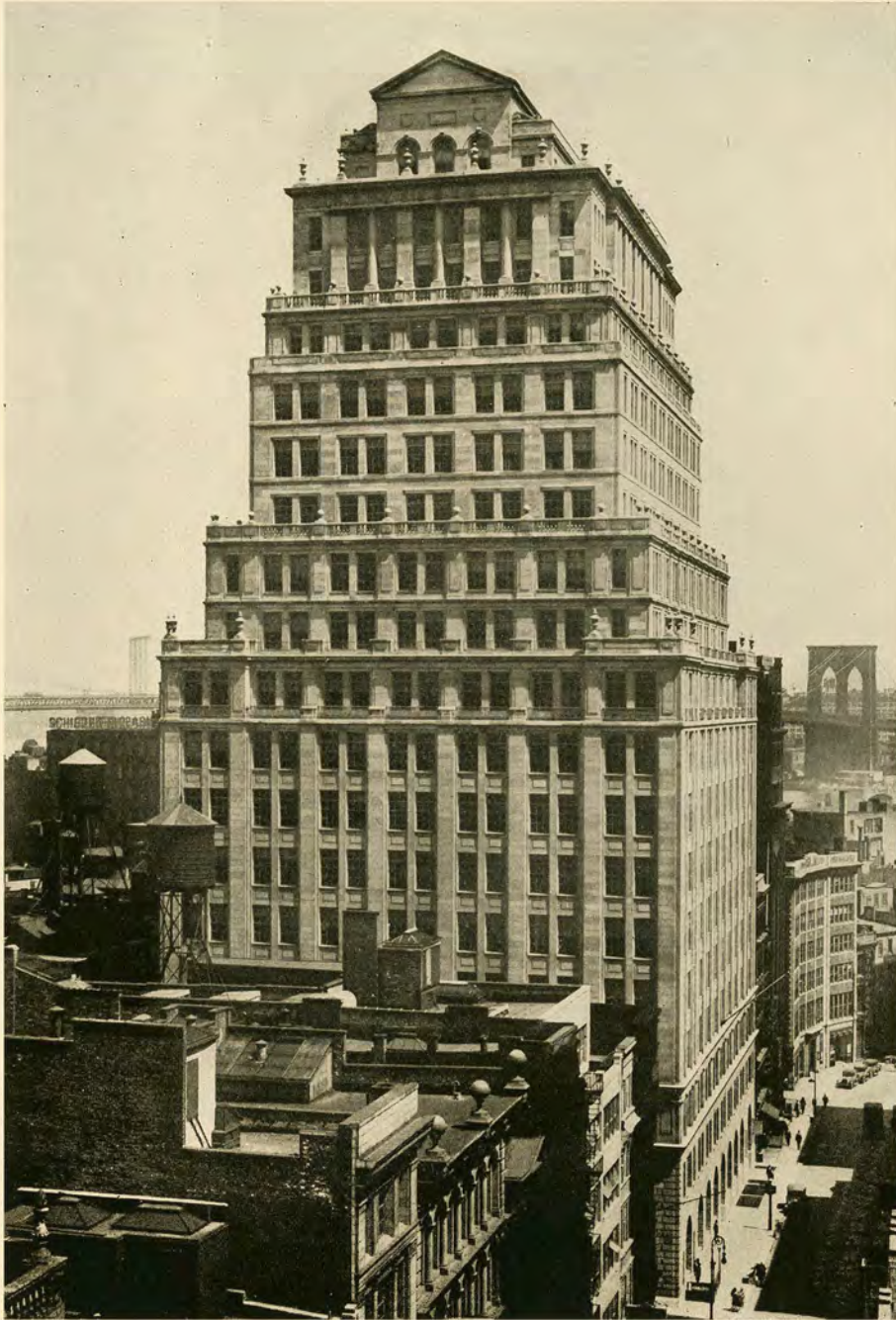
ROYAL INSURANCE CO. BUILDING, NEW YORK Starrett and Van Vleck, Architects
