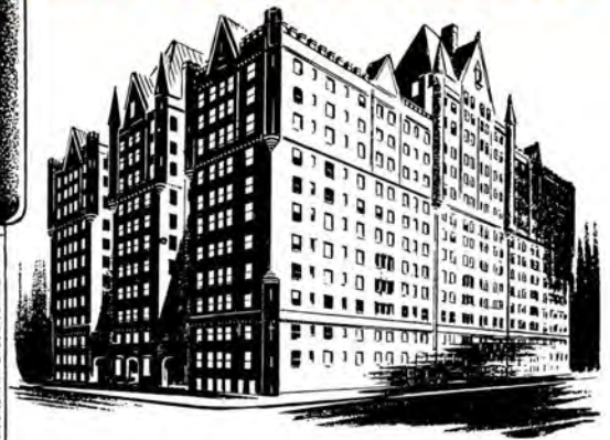
Apartment Building Plumbing and Heating
