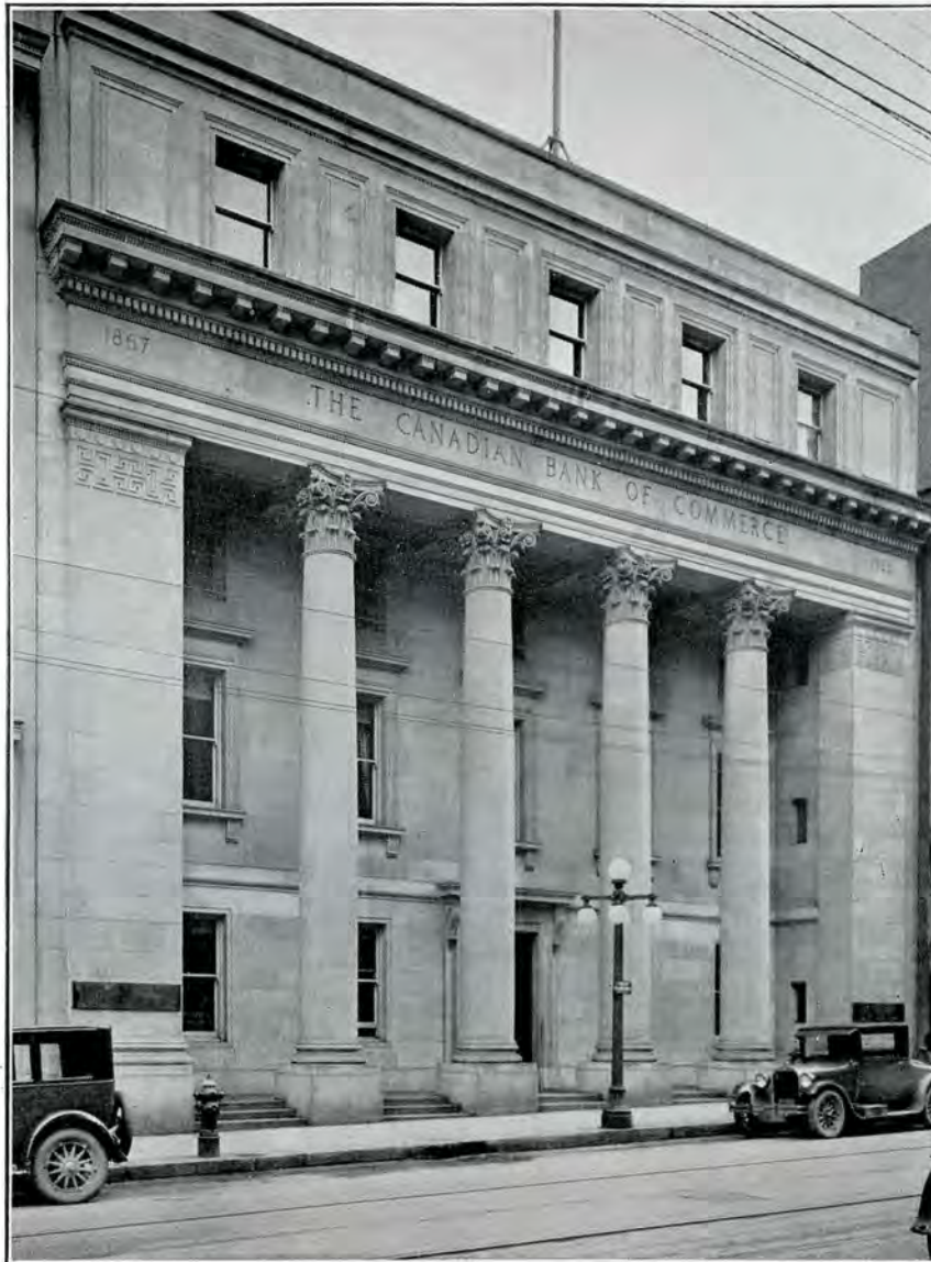
Canadian Bank of Commerce, Ottawa, Ontario. Darling & Pearson, Architects. Built of Gray Indiana Limestone.
