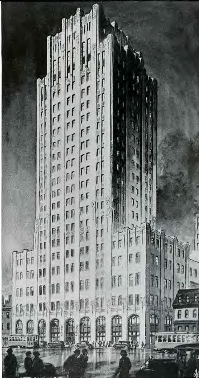
The Toronto Star's New Building Now Being Erected.
