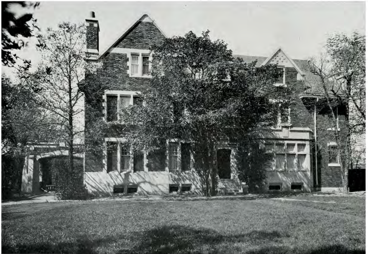
RESIDENCE OF REV. C. W. GORDON, ARMSTRONG'S POINT, MAN. (BUILT 1914) G. W. Northwood, Architect
