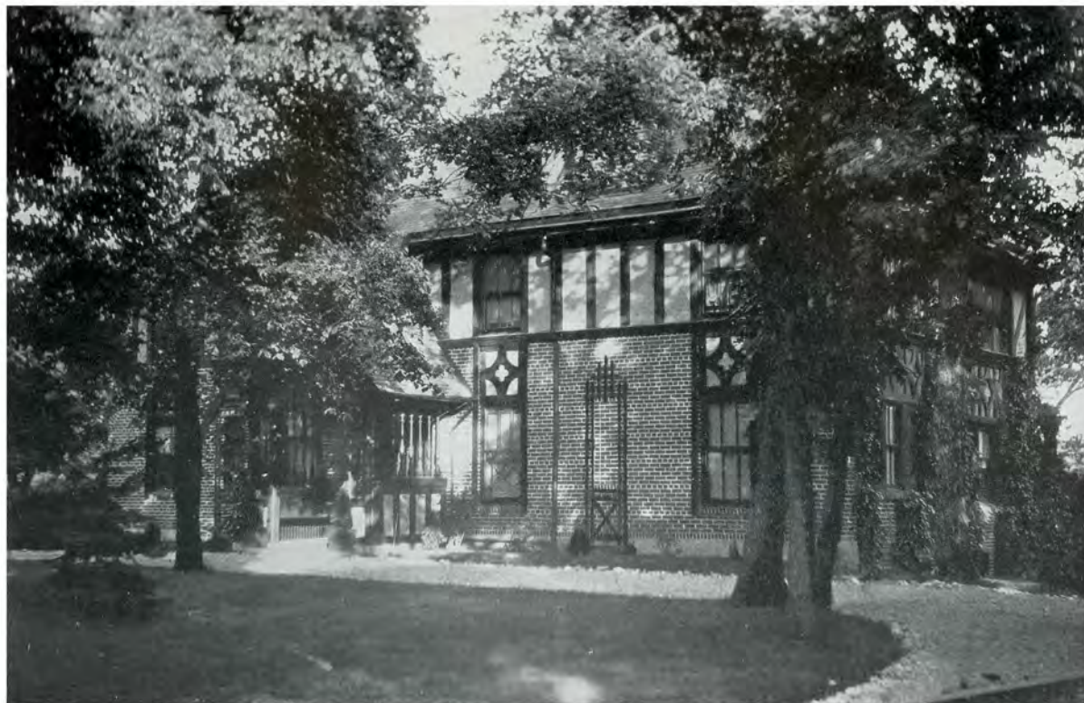
RESIDENCE OF J. H. RILEY, ESQ., ARMSTRONG'S POINT, MAN. (BUILT 1919) Prof. A. A. Stoughton, Architect
