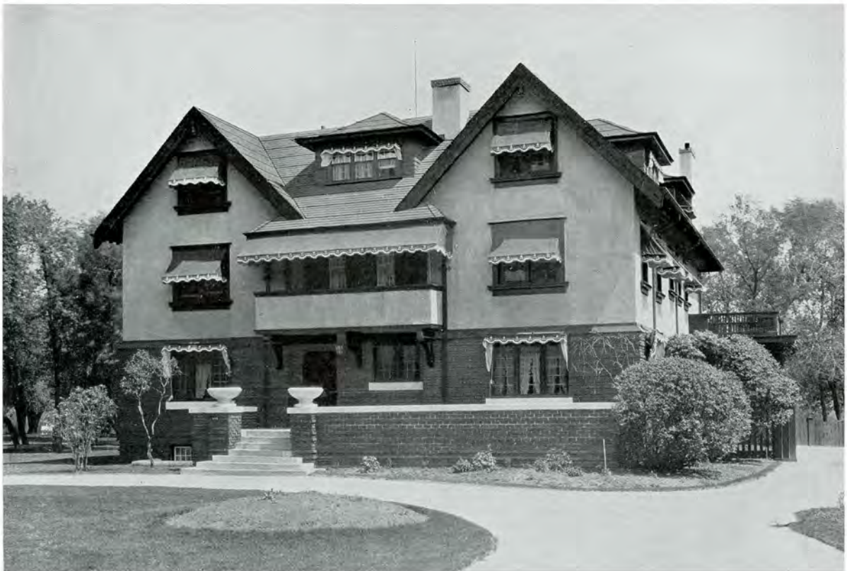
RESIDENCE OF W. A. ANDERSON, ESQ., WINNIPEG, MAN. (BUILT 1912) H. B. Rugh, Architect
