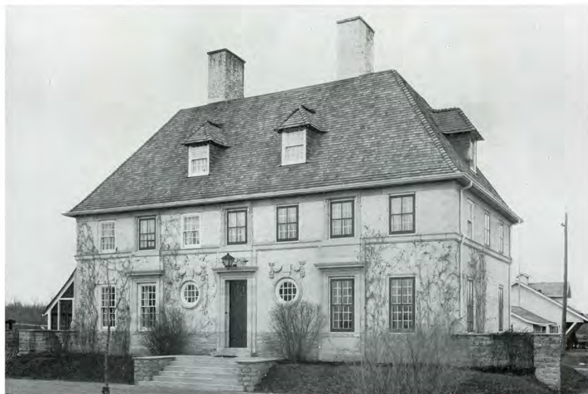
RESIDENCE OF J. H. McDONALD, ESQ., WINNIPEG, MAN. (BUILT 1913) Raymond Carey, Architect
