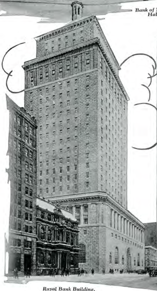
Royal Bank Building, Montreal
