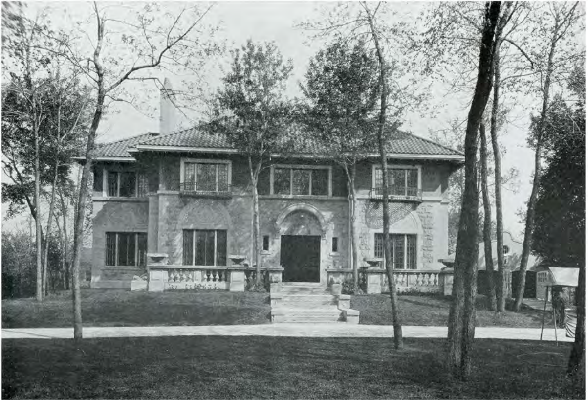
RESIDENCE OF C. G. SPENCER, ESQ., WINNIPEG, MAN. (BUILT 1912) H. B. Rugh, Architect
