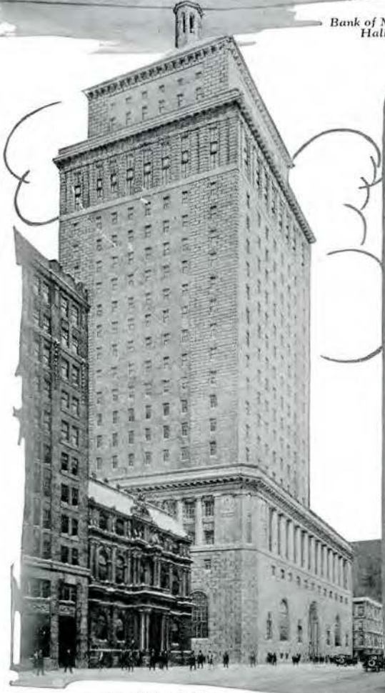
Royal Bank Building, Montreal
