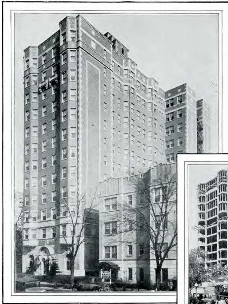
Winthrop Towers Apartments, Chicago. Ground broken April 24, 1927. Building completed in Septem- ber, 1927. (Below) As build- ing looked June 26, 1927, after reinforced concrete frame was completed.
