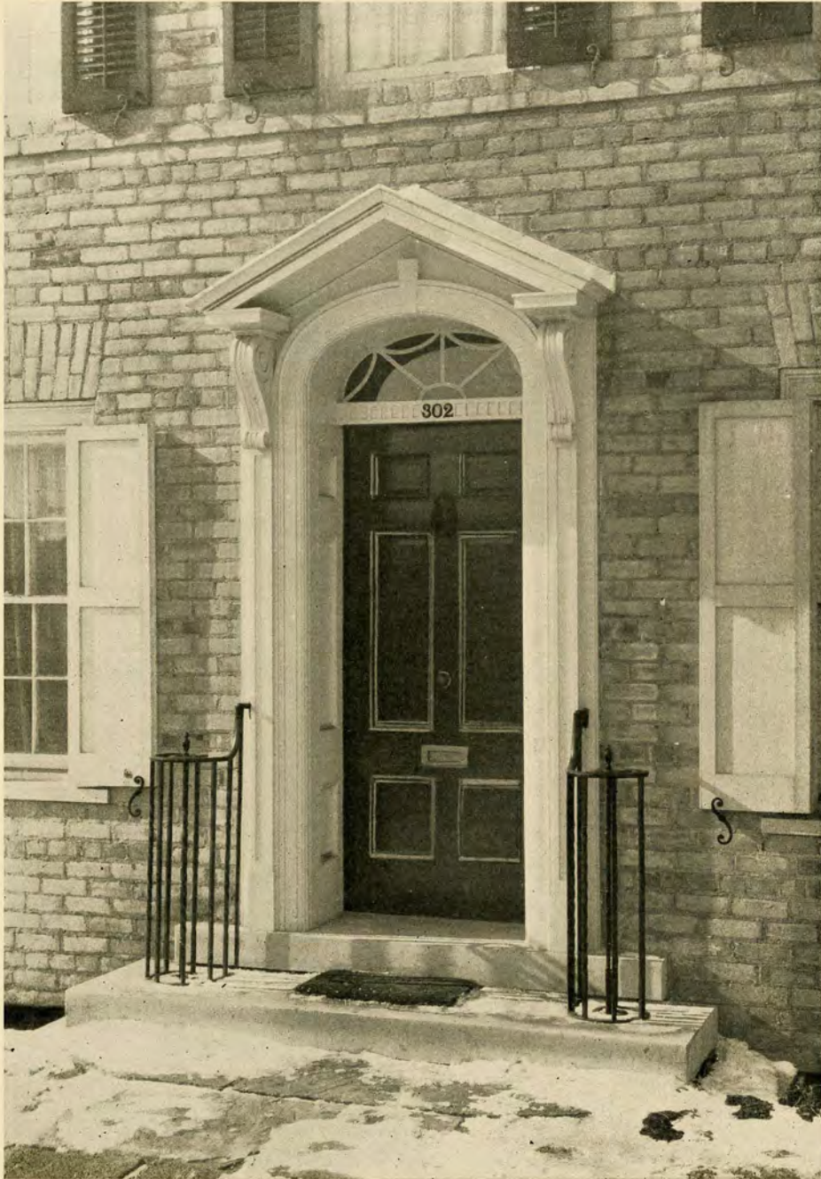
DETAIL OF ENTRANCE, RESIDENCE OF DR. EDWARD MORGAN, TORONTO Dyce E. Saunders, A.R.I.B.A., Architect
