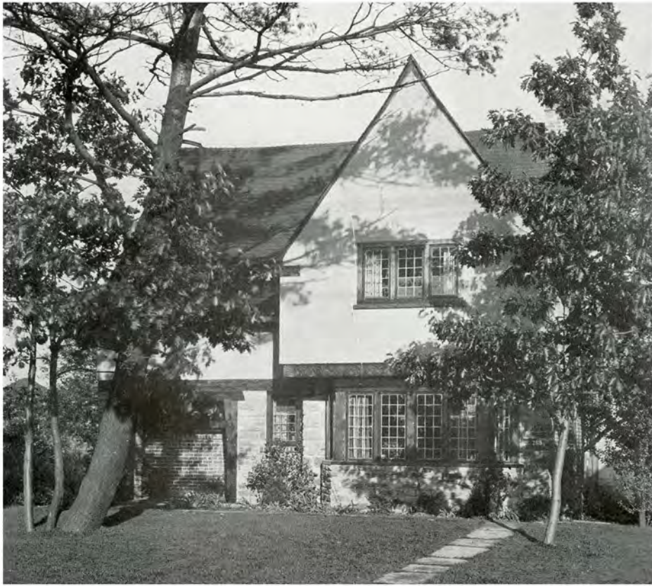
RESIDENCE OF W. L. SOMERVILLE, ESQ., TORONTO W. L. Somerville, A.R.I.B.A., Architect
