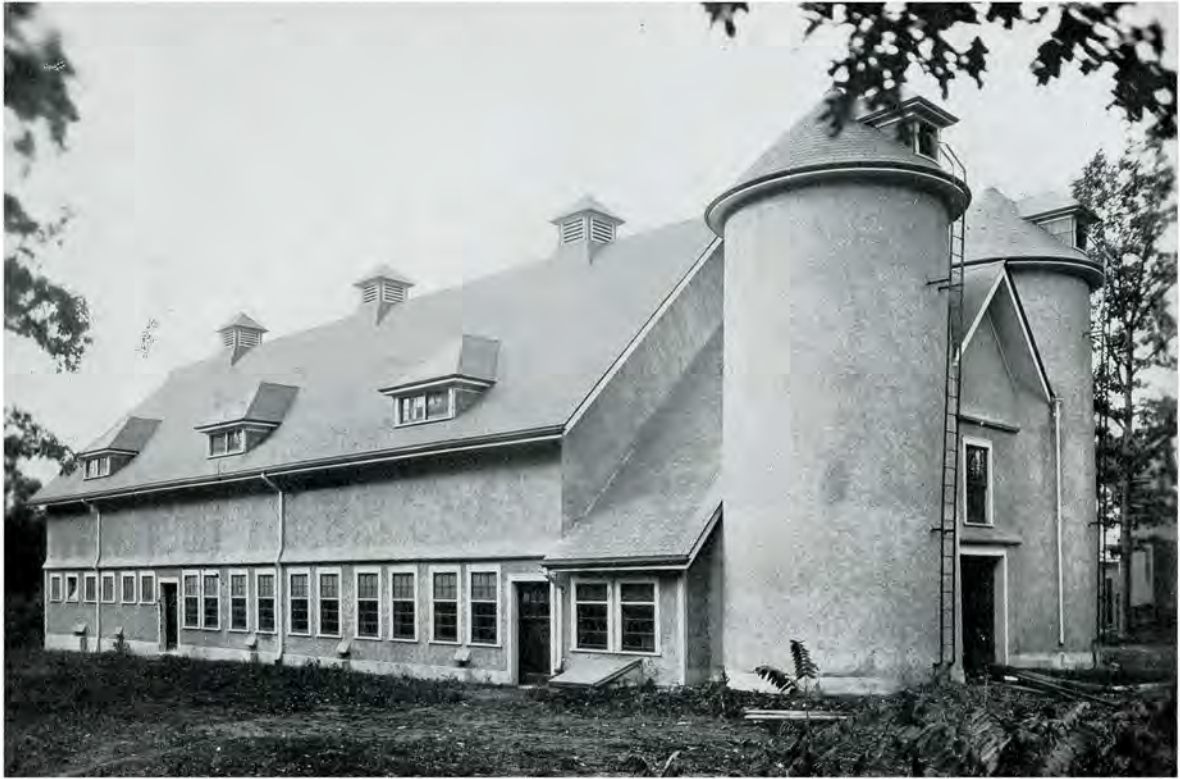
DAIRY CATTLE BARN, SHOWING CONNECTION OF BARN AND SILOS
