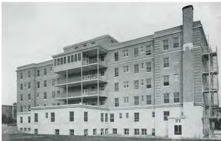
REAR ELEVATION, HOMOEOPATHIC HOSPITAL, MONTREAL Ross & MacDonald, Architects
