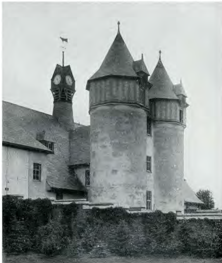
DETAIL OF SILOS, EATON HALL FARM, EVERSLEY, ONT. THE FARM OF LADY EATON Wickson & Gregg, Architects
