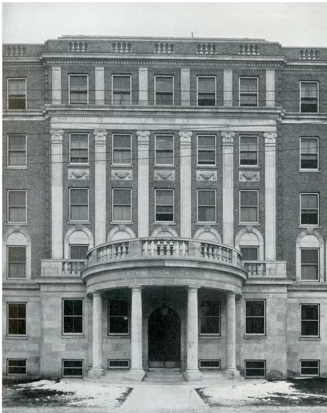
DETAIL OF ENTRANCE BAY—HOMOEOPATHIC HOSPITAL, MONTREAL Ross & MacDonald, Architects
