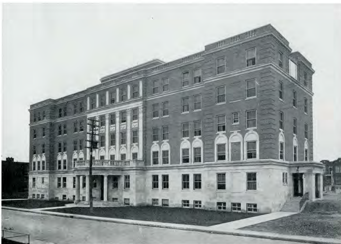
HOMOEOPATHIC HOSPITAL—MONTREAL Ross & MacDonald, Architects
