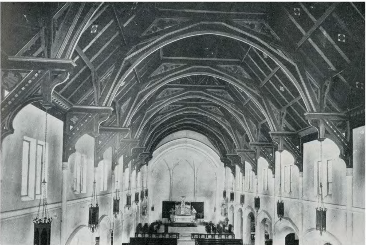
DETAIL OF PANELLED CEILING
