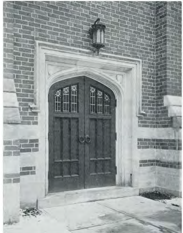
DETAIL OF SIDE ENTRANCE
