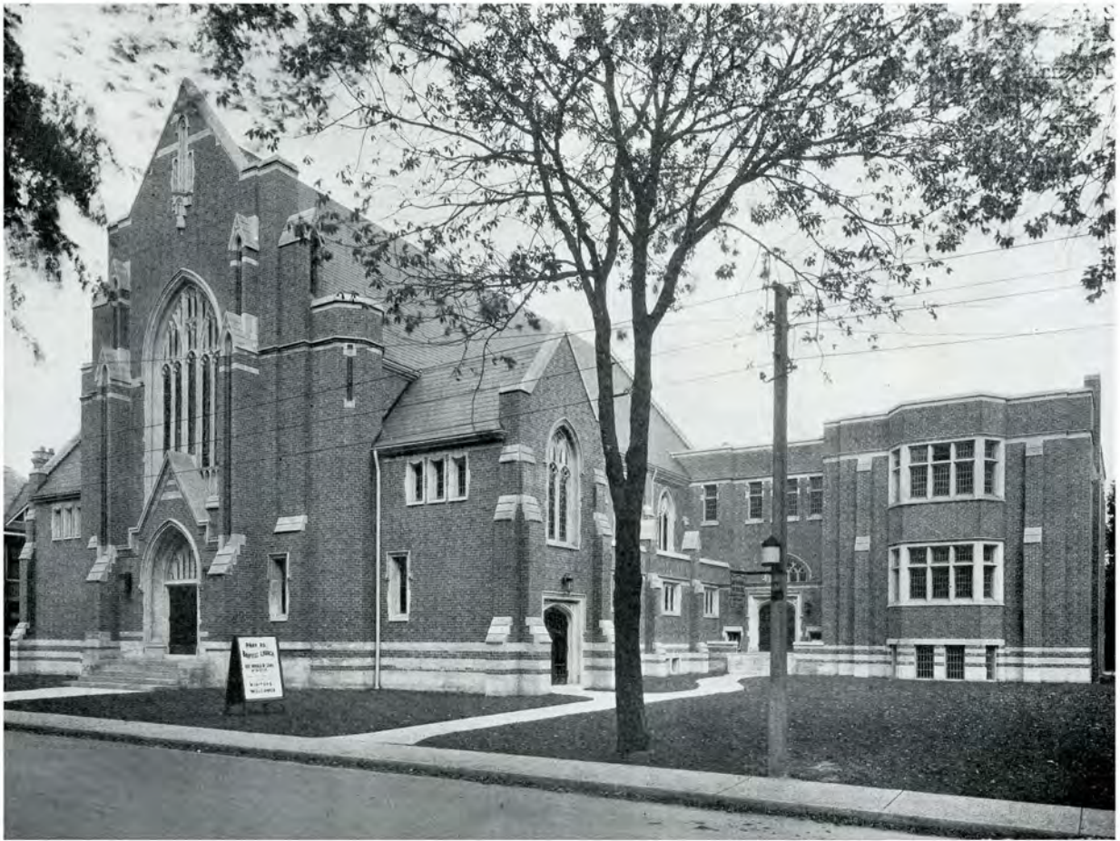
PARK ROAD BAPTIST CHURCH, TORONTO J. Francis Brown & Son, Architects.
