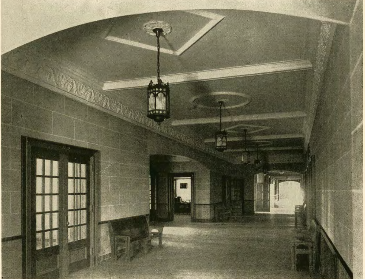
CORRIDOR—RIVERDALE TECHNICAL SCHOOL, TORONTO Architectural Dept., Toronto Board of Education
