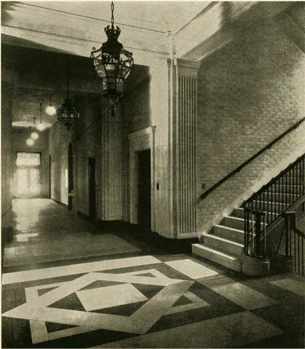
ENTRANCE HALL, HYGIENE BUILDING, UNIVERSITY OF TORONTO Mathers & Haldenby, Architects
