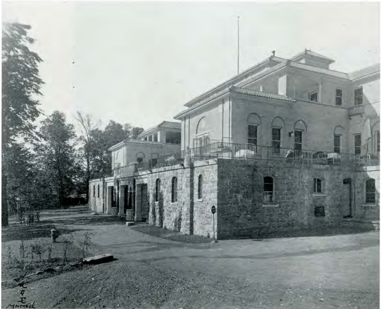
VIEW FROM SOUTH EAST—SHRINERS' HOSPITAL FOR CRIPPLED CHILDREN, MONTREAL, P. Q. J. Melville Miller, R.C.A., and Hugh Vallance, R.C.A., Architects Associated
