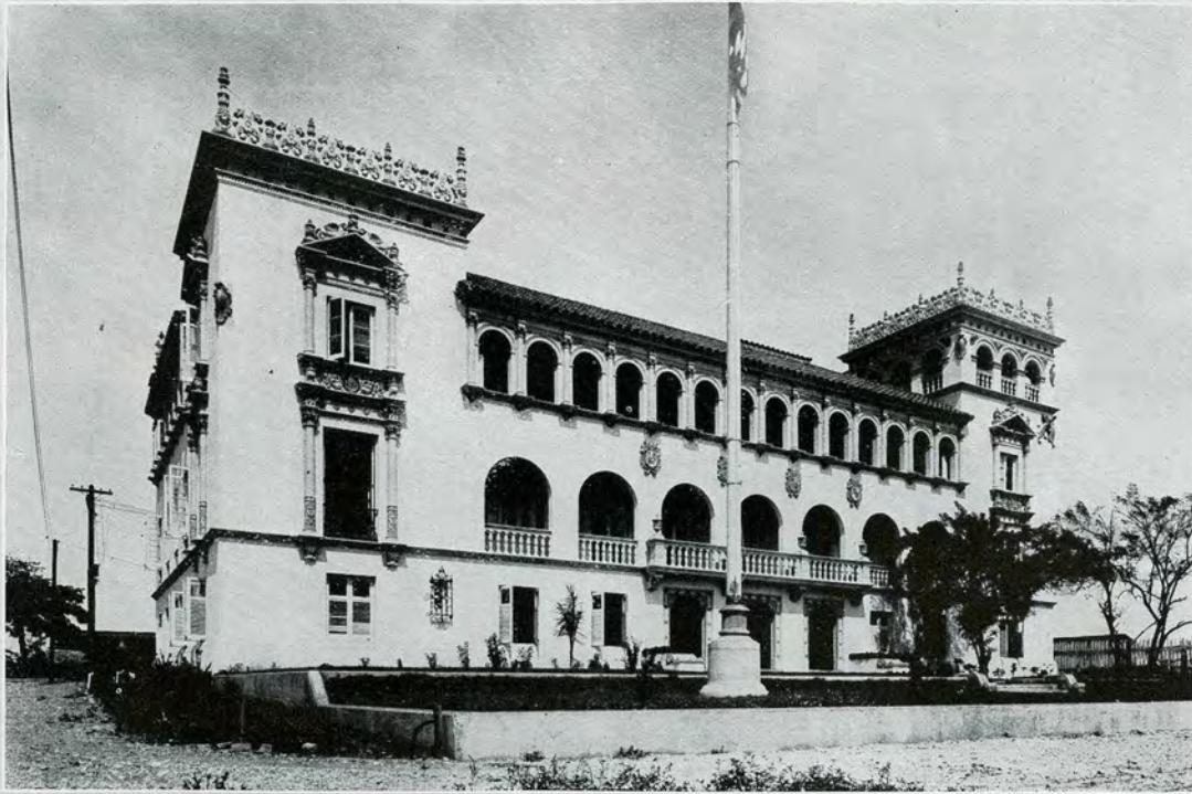
School of Tropical Medicine, San Juan, Porto Rico, Rafael Carmaega, Architect, Teodore Vidal, Builder. Enriched with relief ornamentation in polychrome Terra Cotta
