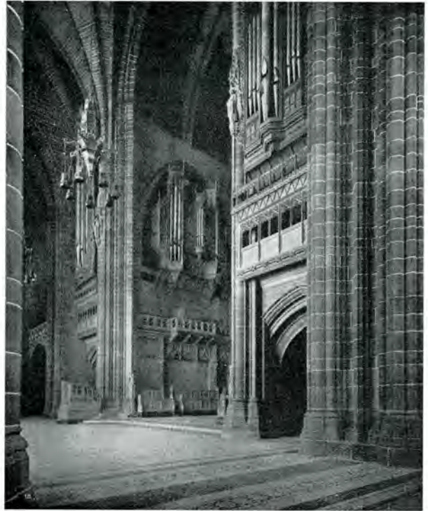
VIEW FROM S. E. TRANSEPT, SHOWING ORGAN, LECTERN, ETC.
