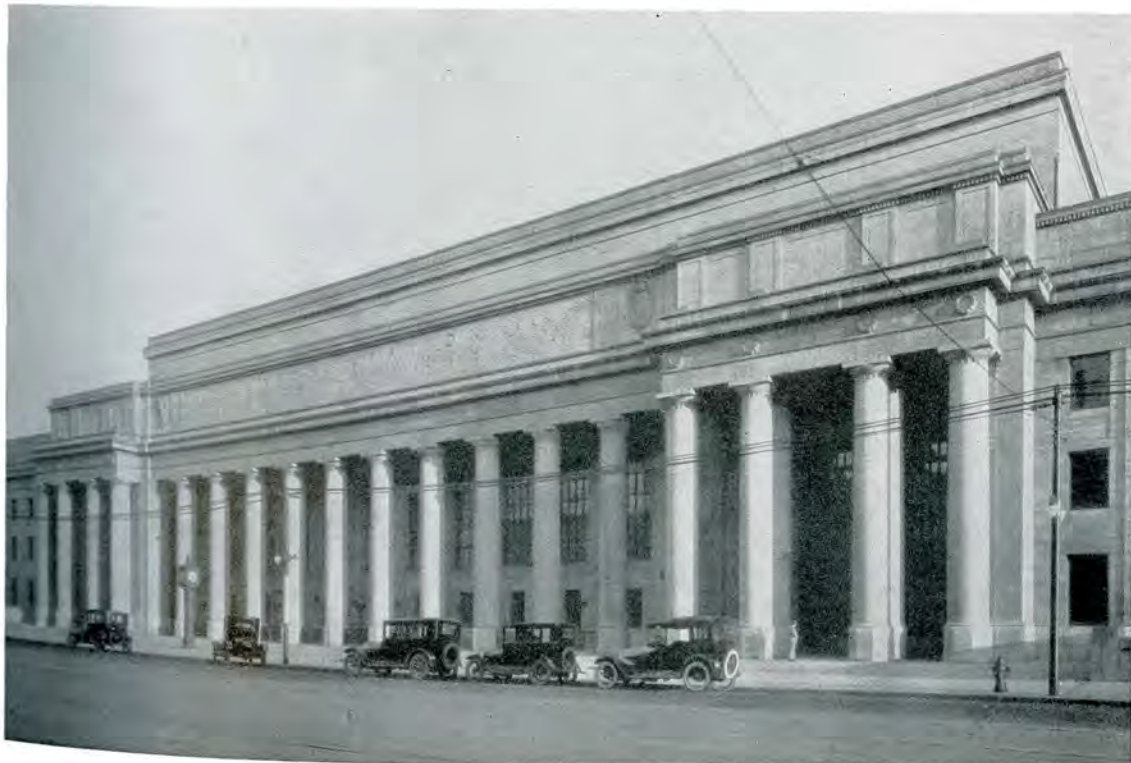
UNION STATION, TORONTO, ONT. Ross & Macdonald, Hugh G. Jones, John M. Lyle, Architects
