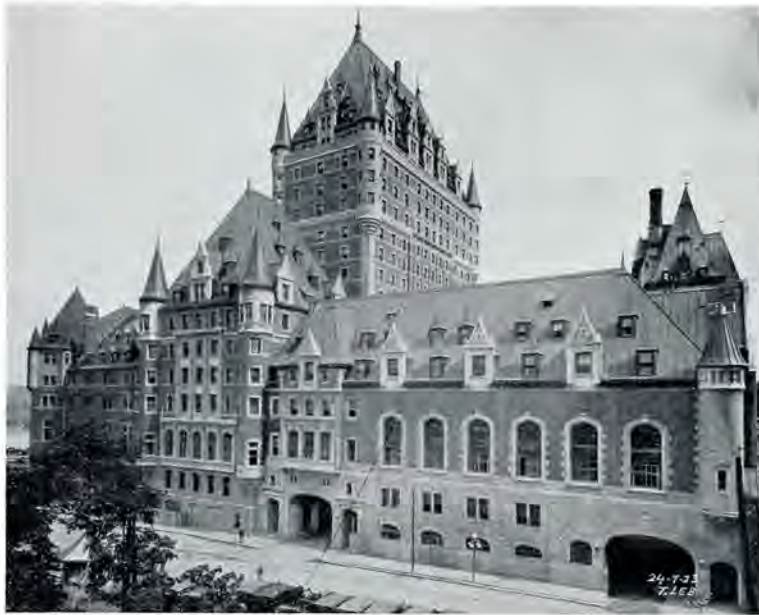
CHATEAU FRONTENAC—VIEW FROM THE SQUARE Bruce Price, Edward & W. S. Maxwell & W. Painter, Architects
