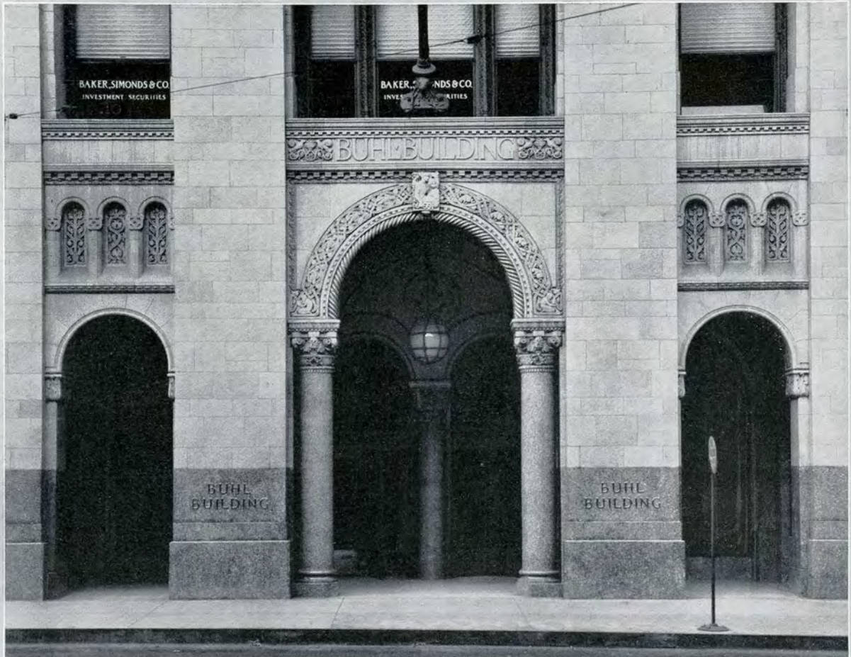
Entrance, Buhl Building, Detroit, Michigan, Smith, Hinchman & Grylls, Architects.
