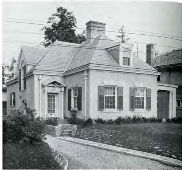
RESIDENCE OF MR. ALLAN ROSS, POPLAR PLAINS ROAD, TORONTO Mathers & Haldenby, Toronto
