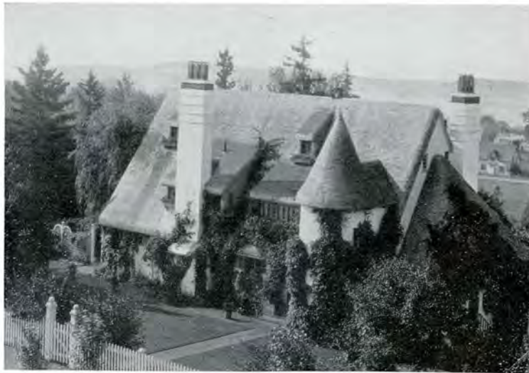
"PANSY-PATCH", RESIDENCE OF MR. HAYTER REED, ST. ANDREWS-BY-THE-SEA, N.B. C. J. Saxe, Architect
