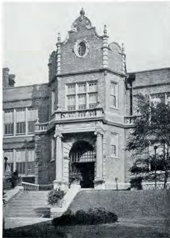
Fig. 6—AN ATTRACTIVE ENTRANCE. COTE BRILLIANTE SCHOOL, ST. LOUIS, MISSOURI. Wm. B. Ittner, Architect
