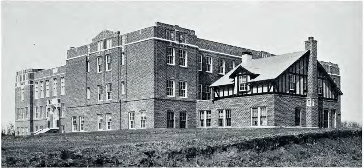
TEACHING AND ADMINISTRATION BUILDING, DORMITORY AND INFIRMARY, CONCORDIA COLLEGE, EDMONTON, ALBERTA. G. H. MacDonald and H. A. Magoon, Architects.
