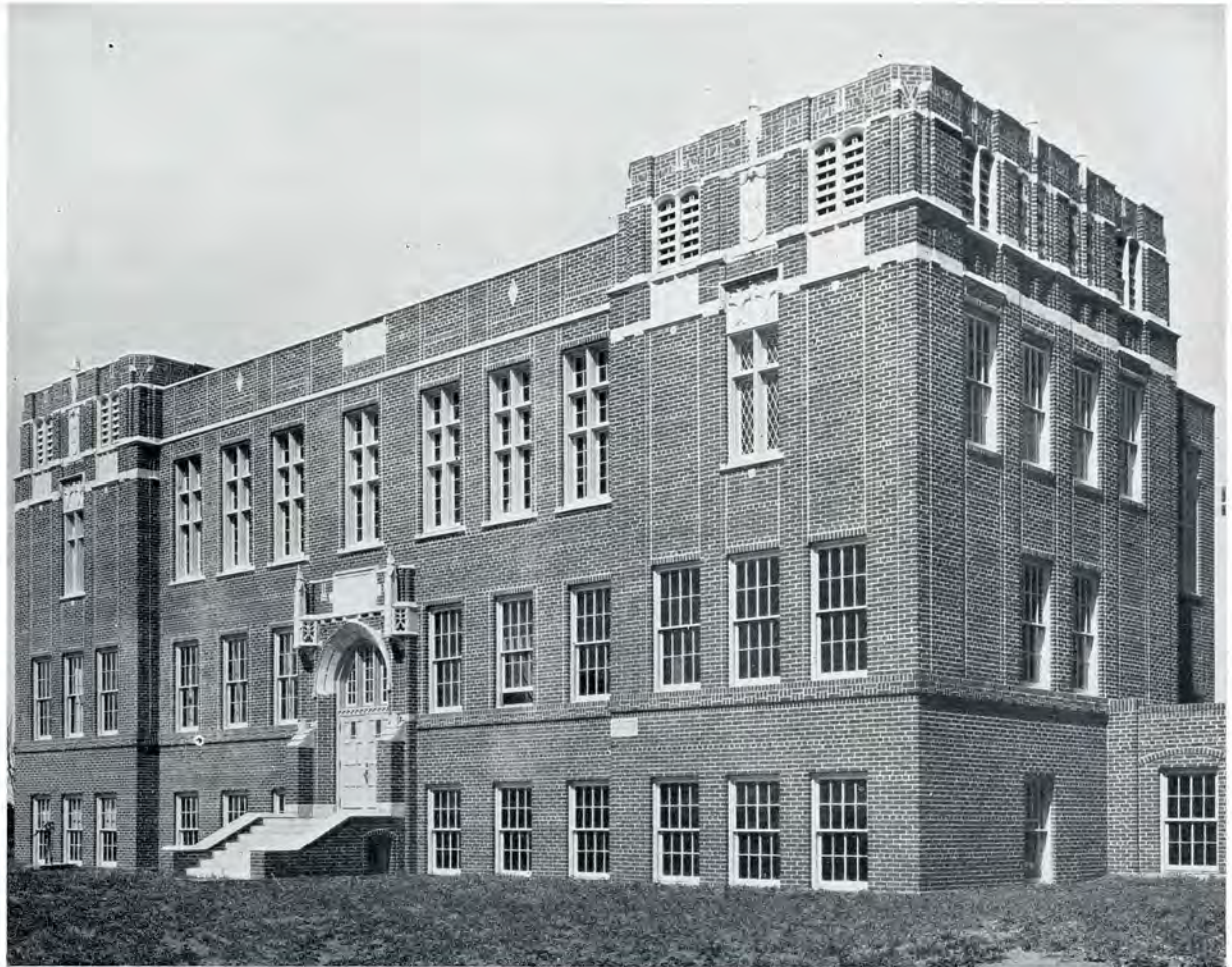
TEACHING AND ADMINISTRATION BUILDING, CONCORDIA COLLEGE, EDMONTON, ALBERTA G. H. MacDonald and H. A. Magoon, Architects.
