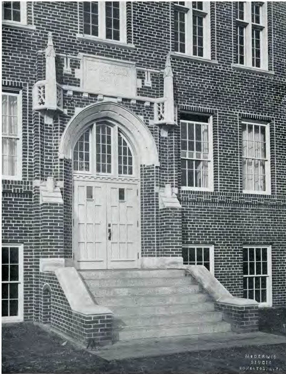
MAIN ENTRANCE, CONCORDIA COLLEGE, EDMONTON, ALBERTA.
