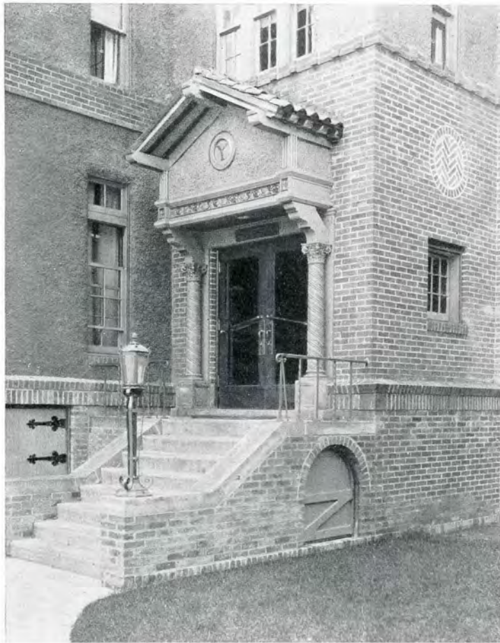
CAFETERIA ENTRANCE, COMBINED Y.M.C.A. AND Y.W.C.A. BUILDING, WINDSOR, ONT. Nichols, Sheppard and Masson, Architects
