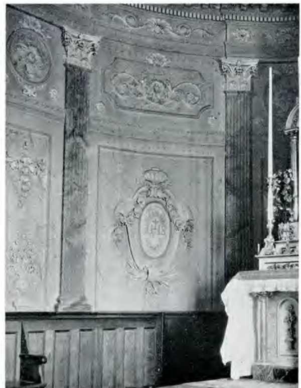
ST. FRANÇOIS—PANELLING ABOVE SIDE ALTARS AND MAIN CORNICE.
