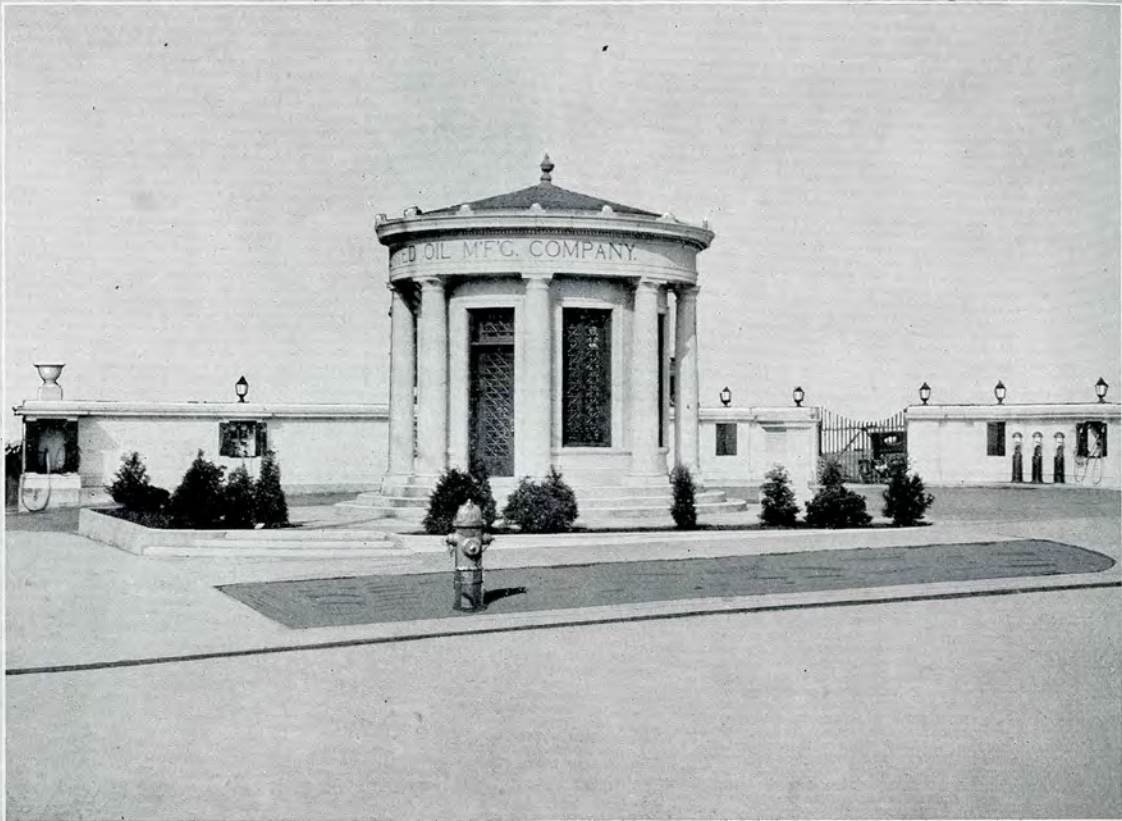
Filling Station for United Oil Manufacturing Company, Eric, Pa. Cody-Hicks-Davidson, Architects. Executed in ivory glazed Terra Cotta with green lettering.
