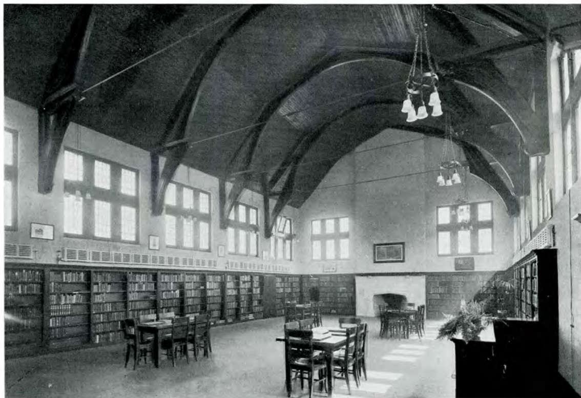
READING ROOM, WYCHWOOD BRANCH, TORONTO PUBLIC LIBRARY Eden Smith & Son, Architects.
