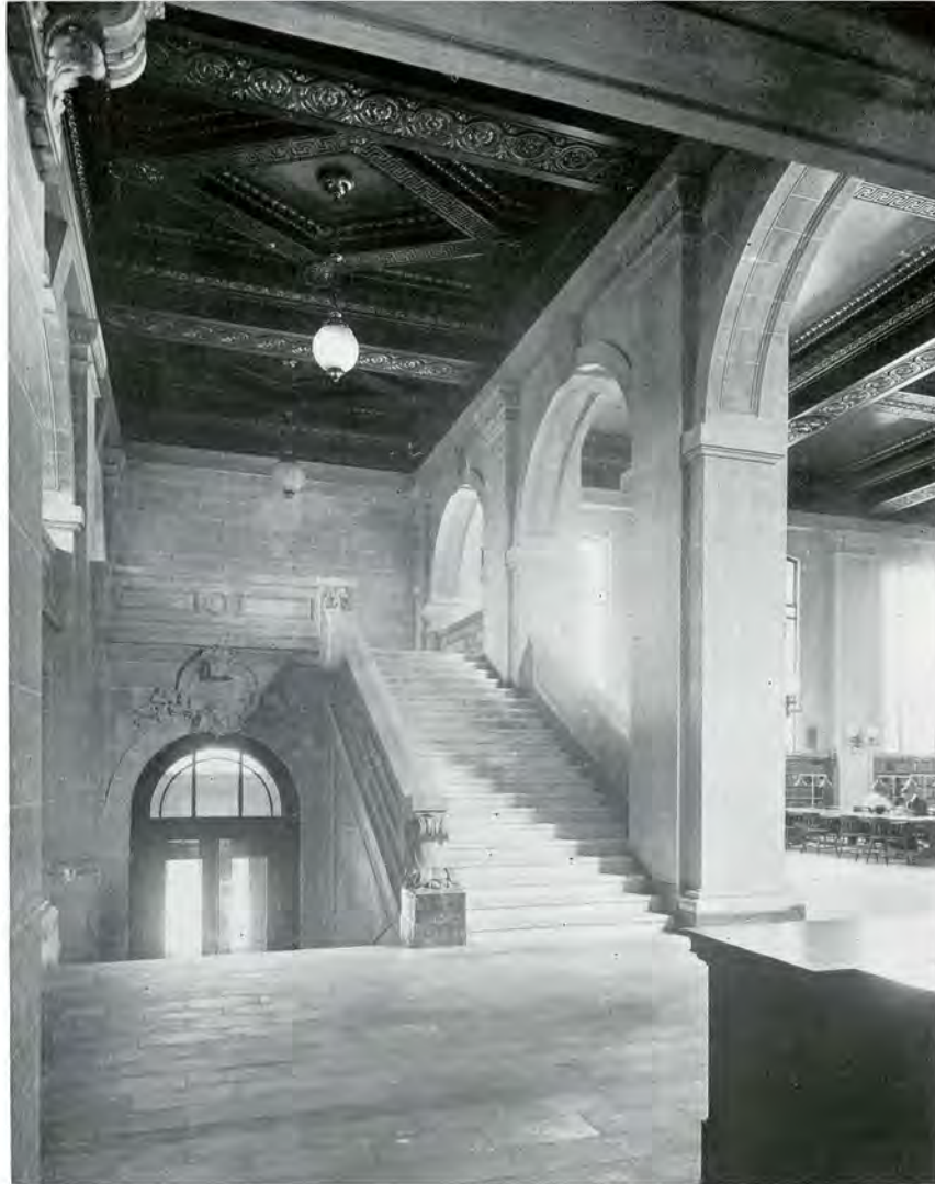
ENTRANCE HALL, PUBLIC LIBRARY, COLLEGE STREET, TORONTO
