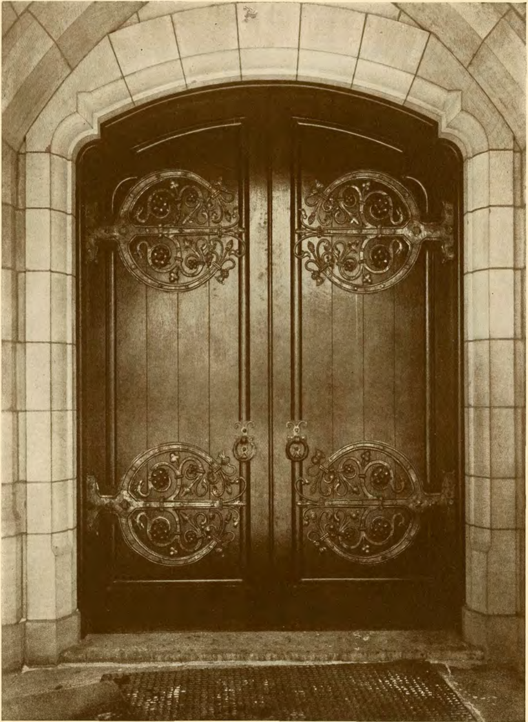
HINGES AND DOOR PULLS ON MAIN ENTRANCE TO SENATE CHAMBER, PARLIAMENT BUILDINGS, OTTAWA
