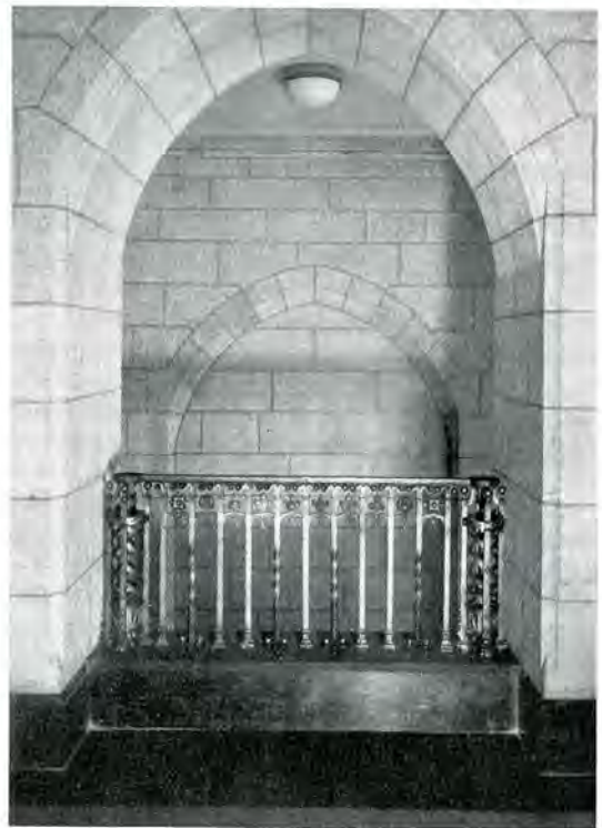
FIG. 5. FORGED IRON RAILING, HEAD OF NORTH STAIRWAY EMBLEMS—TUDOR ROSE, THISTLE, SHAMROCK, FLEUR DE LYS, AND MAPLE LEAF IN CENTRE
