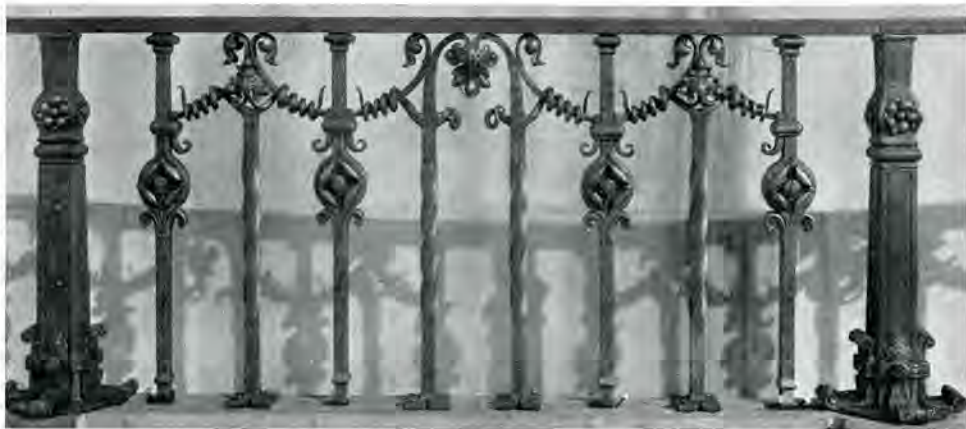
FIG. 6. DETAIL OF WROUGHT IRON RAILING, PARLIAMENT BUILDING, OTTAWA Richard Wright, Chief Architect, Dept. of Public works T. Rankin, Designer Paul Beau, Craftsman
