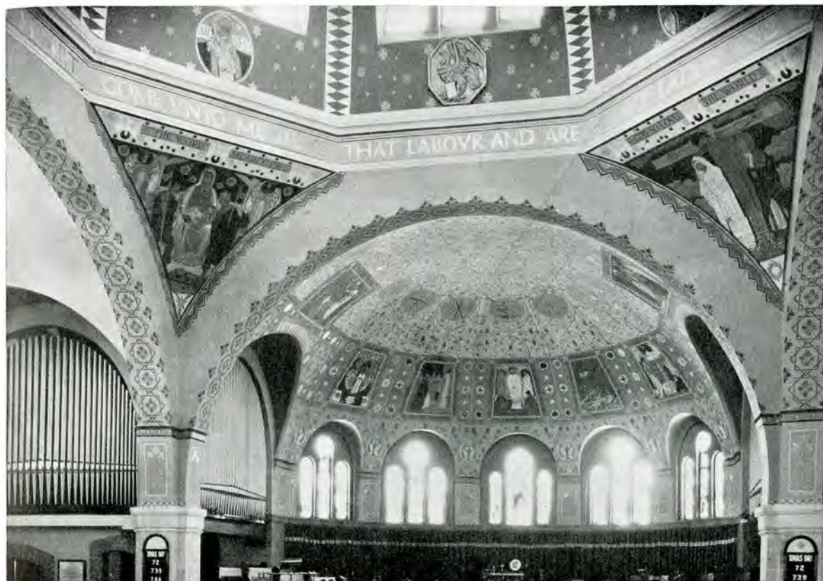
INTERIOR ST. ANNE'S CHURCH, TORONTO, SHOWING CHANCEL, TWO PENDENTIVES AND PART OF DOME
