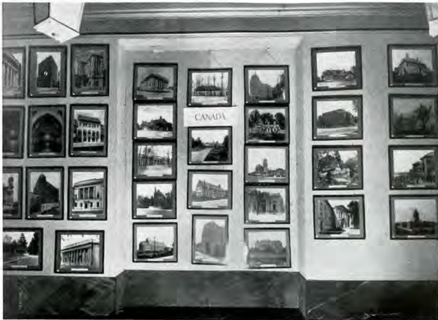
PORTION OF CANADIAN EXHIBIT AT THE ARCHITECTURAL AND ALLIED ARTS EXPOSITION IN GRAND CENTRAL PALACE, NEW YORK
