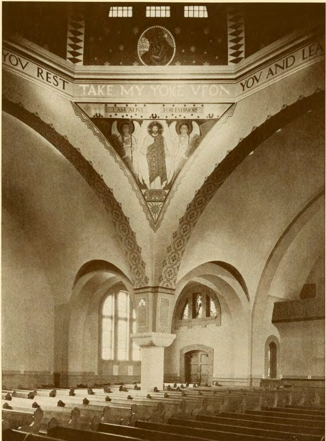
INTERIOR ST. ANNE'S CHURCH, TORONTO. SHOWING PENDENTIVE AND PART OF CORNICE AND DOME Pendentive painting, The Resurrection, by H. S. Palmer, A.R.C.A.
