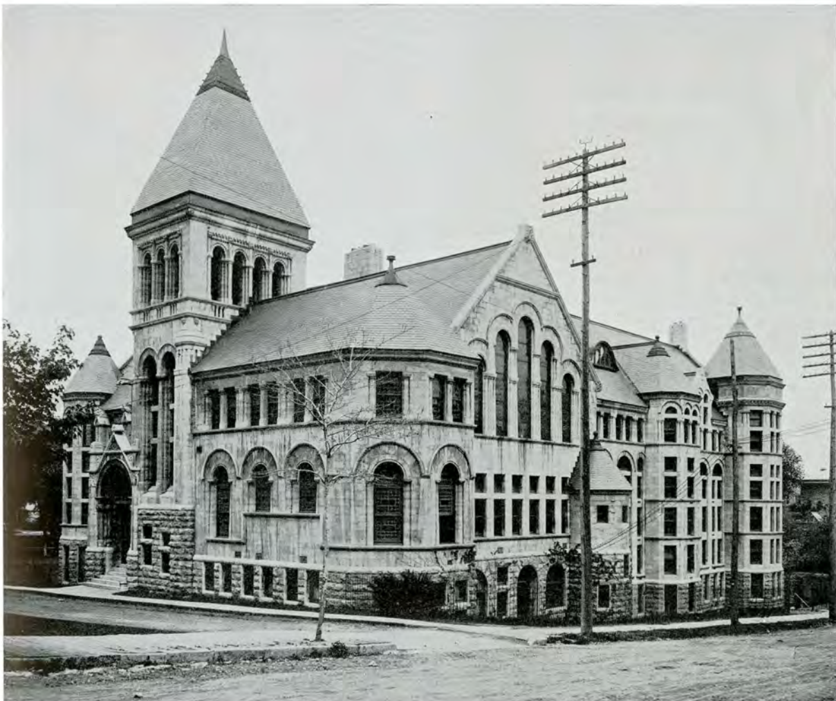
THE REDPATH LIBRARY, MCGILL UNIVERSITY, MONTREAL, 1891 Taylor & Gordon Architects.
