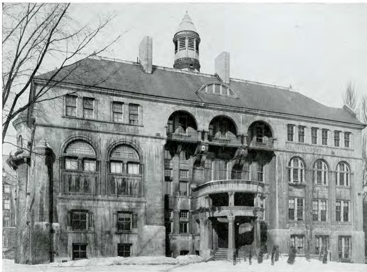
THE MACDONALD PHYSICS BUILDING, MCGILL UNIVERSITY, MONTREAL, 1890 Taylor, Hogle and Davis, Architects
