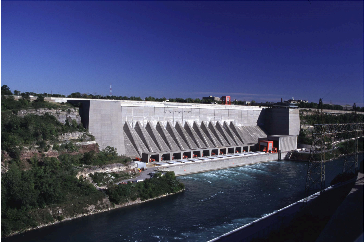
Image 13.5. Hydroelectricity is a renewable source of energy. This facility taps part of the flow of the Niagara River to generate electricity. Source: B. Freedman.
