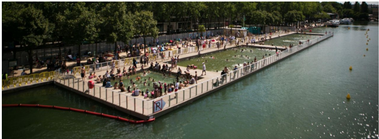
Figure 2 La Baignade dans la Bassin de la Villette (Paris, France). The image shows three pools of varying depth, with nearby change rooms, showers, and bathrooms. Designed by Patrick Charoin + Marina Donda, architects.
