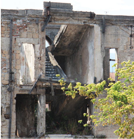
Ruin: An abandoned apartment block in Mostar, BiH
