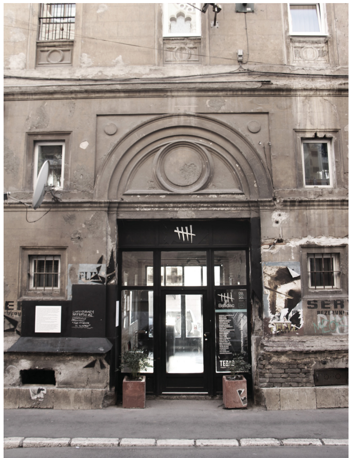
Brodac Gallery rebuilt among the ruins of the Beledija Building in Sarajevo
