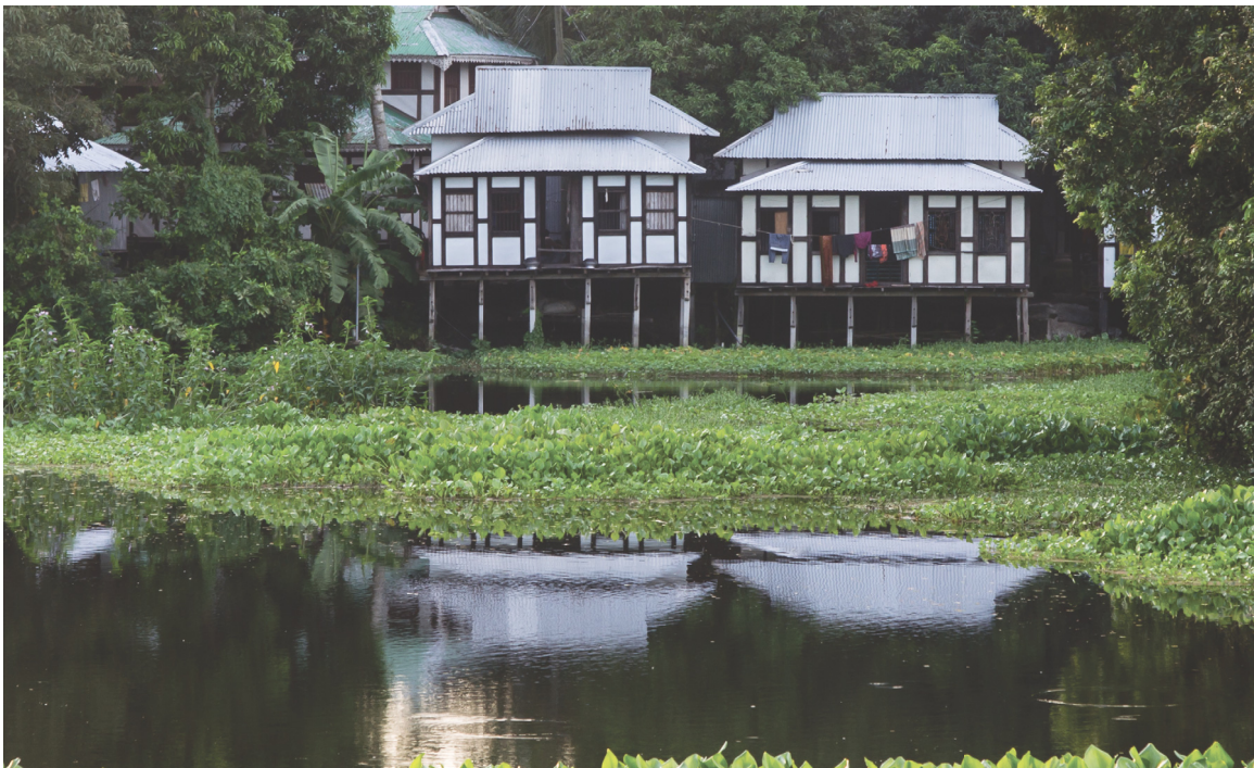
Fig 11: Homes with half a floor on top for dry storage in Shreenagar
