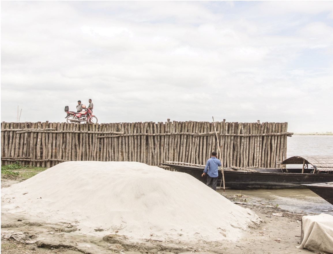
Fig 4: Photograph of a dock structure in Gaibandha
