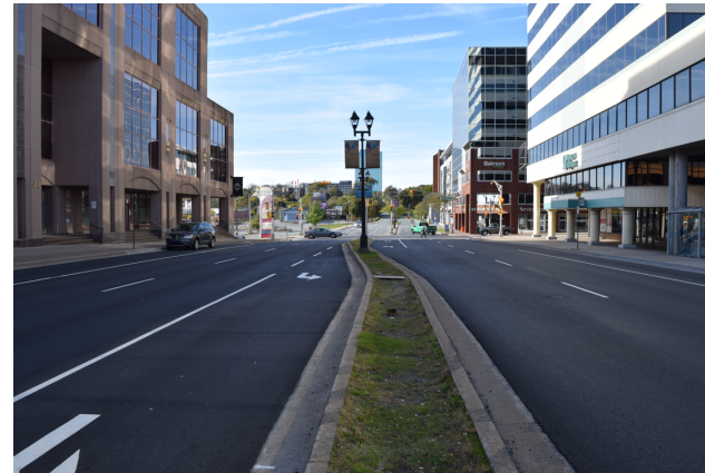
Figure 2.9: Alderney Drive at Queen Street (looking west)
