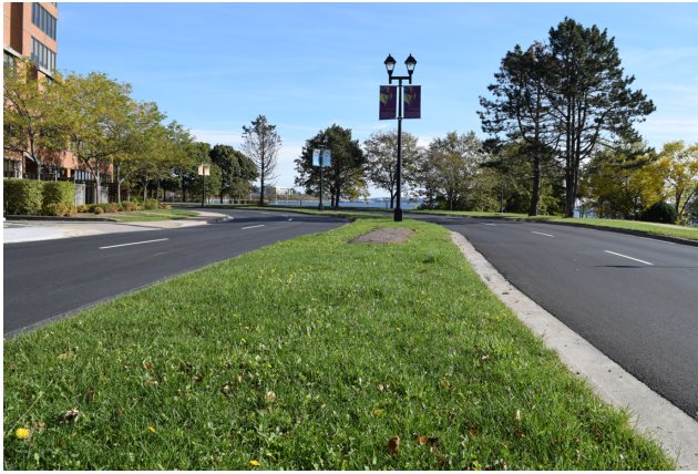
Figure 2.10: Alderney Drive at Portland Street (looking east)
