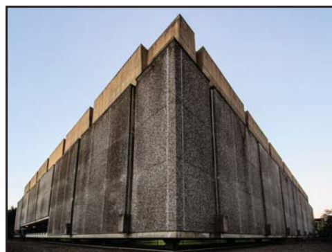
Fig. 34. Leslie R. Fairn, Killam Memorial Library, 1966-71. The use exposed aggregate concrete panelling is characteristic of brutalist structures.
