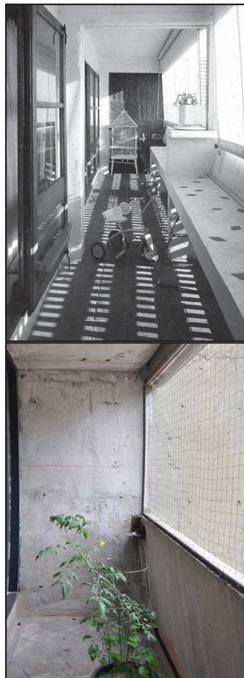
Fig. 61. and 62. Residential tower balconies. Above: The balconies of Unité d'habitation at Marseille; from Jenkins, Unité d'Habitation: Marseilles . The Unité provides greater environmental control to tenants. Use of concrete brise-soleil, blinds, and cross-unit ventilation help to mitigate the heat of summer months, while enhanced habitability of the balcony allows the living areas to expand outdoors, and favorable outdoors conditions to permeate the interior space. Below: The balconies of Fenwick Place are much smaller and provide much less desirable conditions for habitation. The added environmental buffer that was capitalized in the prototype has been reduced to wire mesh screens that prevent birds from roosting and tenants from throwing items in protest.
