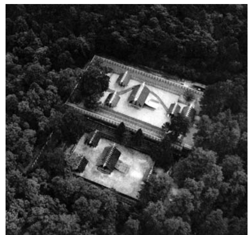
Fig. 93. and 94. Ise Grand Shrine , 640 BCE; photograph from Yamato People; diagram by author. Shown halfway through renewal process, the old shrine at the bottom is about to be dismantled and the site left blank for the next twenty years.
