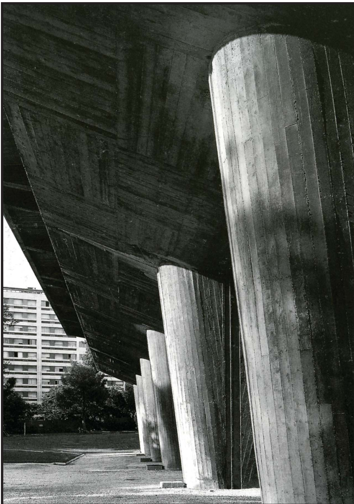
Fig. 51. Photograph of the pilotis of the Unité d'habitation in Marseille, a consistent feature of Le Corbusier's residential schemes. Departing from earlier expressions, at the Unité the pilotis evince the materiality of concrete, the texture of the cast-in-place process of construction, are heroic in their scale, while at the same time humanized by the organic taper of their form. These attributes in part inspired the brutalist movement; Photograph by David Jenkins, from Unité d'Habitation: Marseilles .
