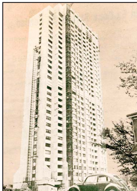
Fig. 53. Fenwick Place under construction; from 4th Estate October 15, 1970.
