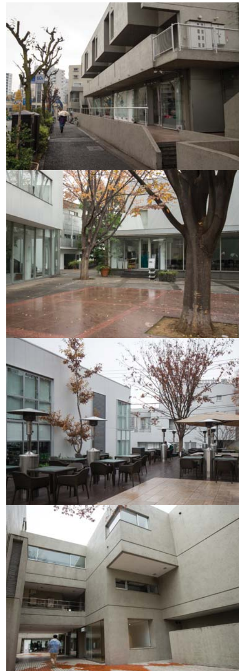
Fig. 111., 112., 113., and 114. Fumahiko Maki, Hillside Terrace , 1969-1992; photographs by Evan Chakroff, from Flickr. Photographic sequence showing the various links in between buildings that create a successful groupform over time.
