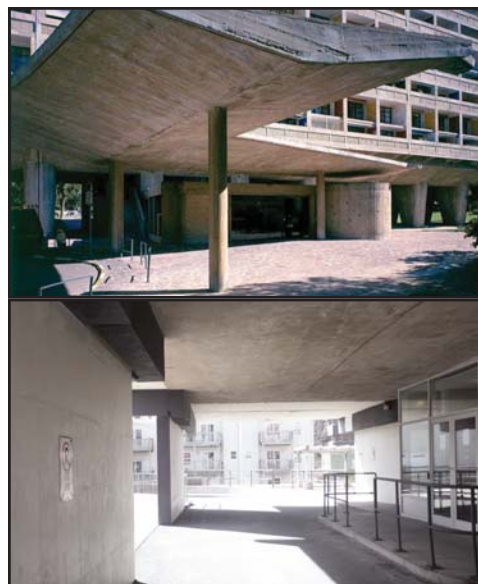
Fig. 74. and 75. Residential tower entrance. Above: The porte-cochère of the Unité d’habitation ; from Fondation Le Corbusier. The entry of the Unité is both sculptural and links the building to existing pedestrian paths and boulevard. Below: The porte-cochère at Fenwick Place, connects entrance to a private driveway off of Fenwick Street.
