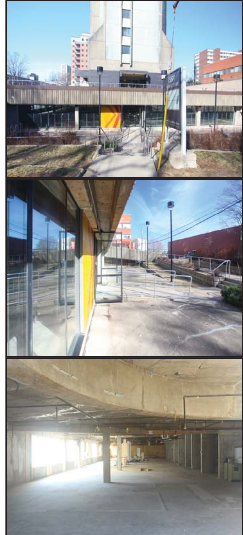
Fig. 79. Series of photographs showing the sequence of spaces leading to the commercial space on the ground floor, which is currently vacant.
