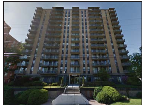
Fig. 38. Macdonald Apartments, 1971. 14-storeys tall.
