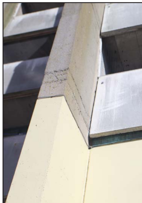
Fig. 6. Fenwick's un-faced concrete cladding and structure.
