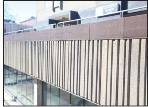
Fig. 55. Precast concrete panels with exposed aggregate finish and recessed texture, used at plinth level to enhance brutalist materiality and humanist expression.
