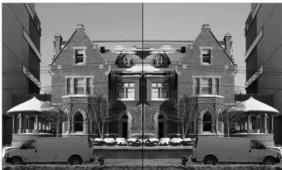
FIG. 19. THE BLAIKIE AND ALEXANDER HOUSES AT 404 JARVIS STREET, BY ARCHITECTS GUNDRY AND LANGLEY, CONSTRUCTED BY SMITH AND BURKE, 1864 (SHOWING THE UNALTERED LEFT PORTION OF THE HOUSE MIRRORED TO REPLACE THE CURRENT ELEVATION WHICH WAS LATER ALTERED.) THIS BUILDING IS THE EARLIEST REMAINING SEMI-DETACHED EXAMPLE OF THE BAY-AND-GABLE IN TORONTO. | SCOTT WEIR, 2015.
