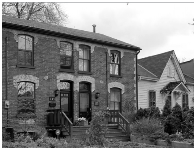
FIG. 26. IMMEDIATE PREDECESSORS OF THE BAY-AND-GABLE IN CABBAGETOWN, THE LATE GEORGIAN ROW-HOUSE TYPE AND THE GOTHIC COTTAGE: 134-136 AMELIA STREET (1884) AND 138 AMELIA (1878). ALTHOUGH NEARLY IDENTICAL IN PLAN TO A BAY-AND-GABLE, 134-136 HAVE THE FLAT FAÇADE OF AN OLDER HOUSE. | SCOTT WEIR, 2015.
