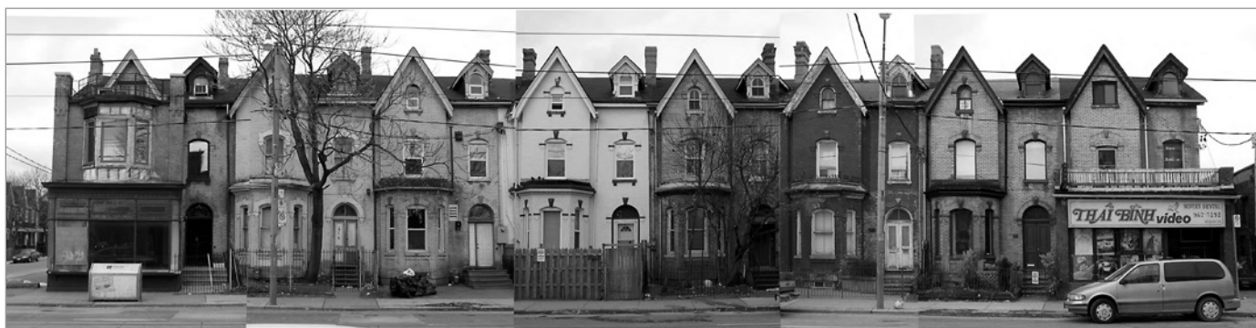
FIG. 25. A ROW OF EIGHT SUBSTANTIAL HOUSES AT 410-432 DUNDAS, 1884, CONSTRUCTED IN SERIES RATHER THAN PAIRED MIRROR IMAGE UNITS. | SCOTT WEIR, 2015.
