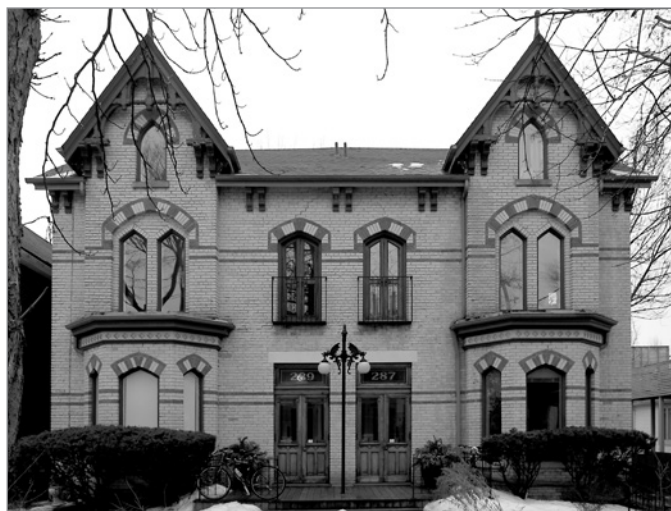
FIG. 28. AN EARLY POLYCHROMY PAIR COMPRISED OF WHITE BRICK WITH RED DECORATIVE ELEMENTS AT 287-289 CARLTON, 1878, BOTH CONSTRUCTED FOR CHRISTOPHER WILSON. BY THE MID-1880S, THE MORE COMMON PALETTE WOULD BECOME RED BRICK FIELD WITH WHITE BRICK DETAILS. | SCOTT WEIR, 2015.
