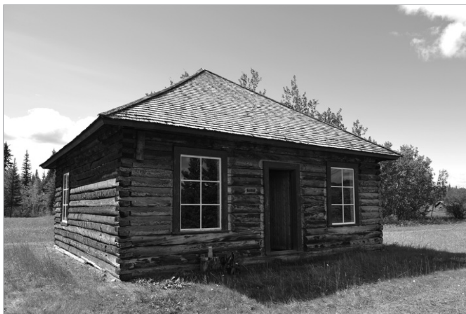
FIG. 22. YUKON FIELD FORCE BUILDING, FORT SELKIRK, 1898. | EMILY TURNER.
