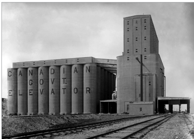
FIG. 2. CANADIAN GOVERNMENT GRAIN ELEVATOR AT OGDEN, ALBERTA (1911), ILLUSTRATED IN LE CORBUSIER, VERS UNE ARCHITECTURE (1923, CHAMPS-FLAMMARION). | PHOTOGRAPH COURTESY OF PROVINCIAL ARCHIVES OF ALBERTA, HARRY POLLARD ARCHIVES.
