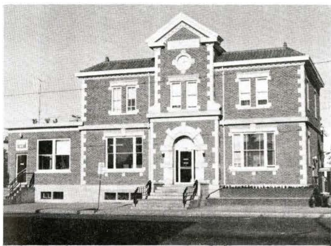
Vegreville Public Building, 1929 Arch.: T.W. Fuller, Jr.
