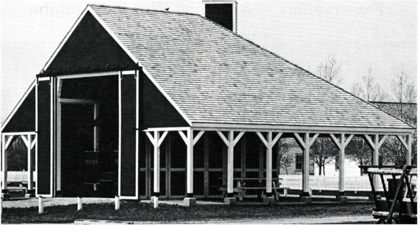
Rudy Friesen's design for the tractor shelter received an Honourable Mention award in the Manitoba Premier's Awards for Design Excellence and was a finalist in the Governor General's Medal for Architecture program.
