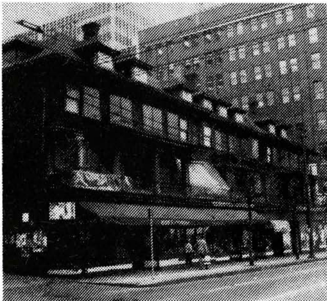
Figure 17. The Orillia, circa 1903, was reduced to rubble in May, 1985 to make way for a planned 16 storey office tower.
