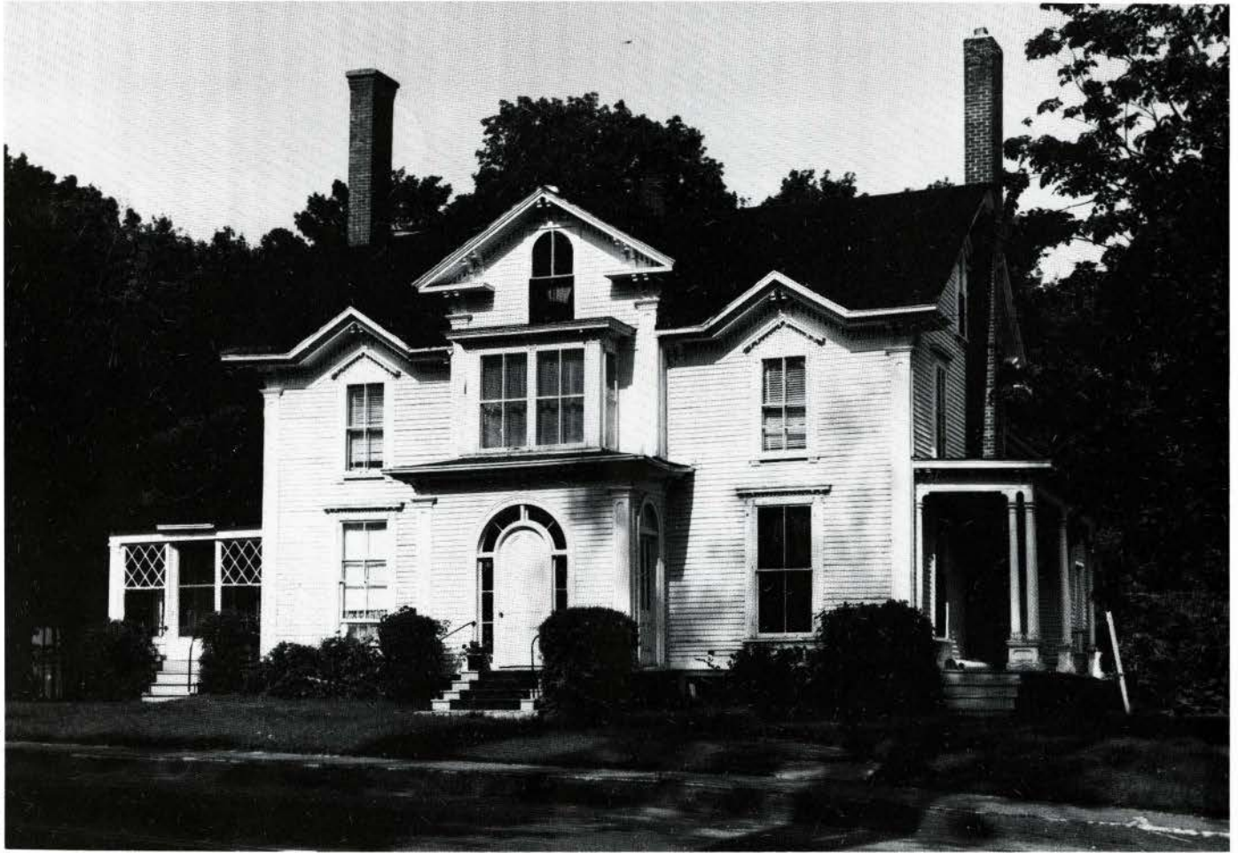
Figure 10. 51 Grove Street, Danville.
