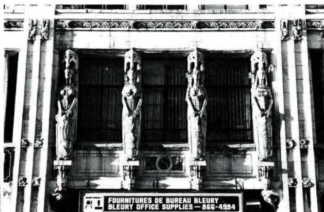
Fig. 9. Southam Building, 1070, rue de Bleury, Montreal; 1913-1914, Brown & Vallance.
