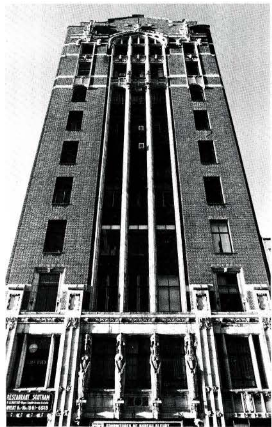
Fig. 10. Southam Building, 1070, rue de Bleury, Montreal; 1913-1914, Brown & Vallance.
